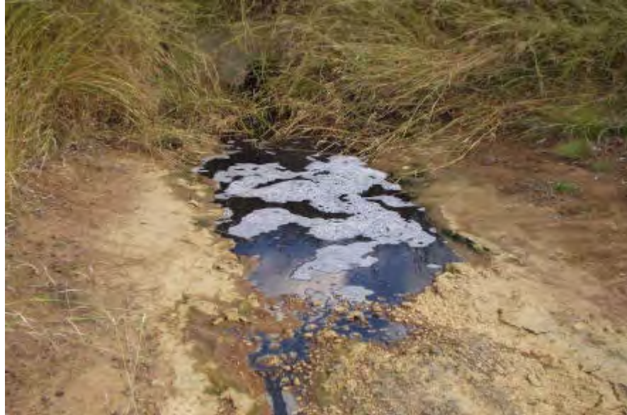
Figure 4.6. Foam waste-water leaking from a collection pit drain within Defence land (RAAF Amberley).
