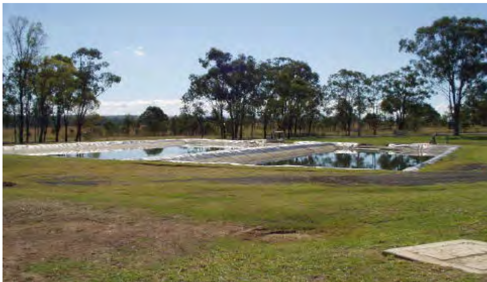
Figure 4.12. AFFF collection pond (left) and water collection pond (right).
