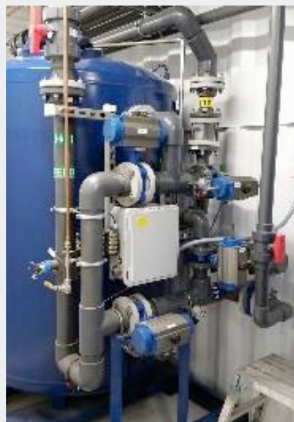
Water treatment plant contained in two shipping containers (above and left)
