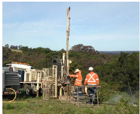
Groundwater bore drilling in the area surrounding HMAS Albatross
