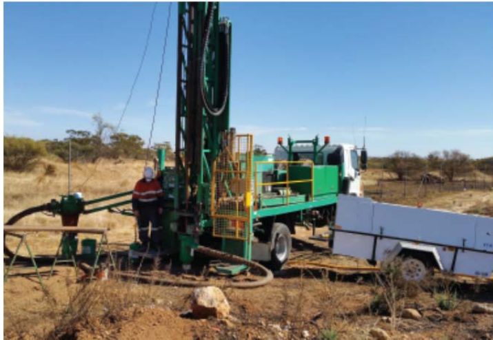
Drill rig used to develop boreholes
