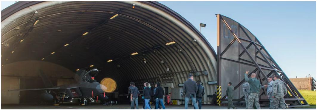
Figure 4: USAF F-22 in hardened aircraft shelter at Spangdahlem, Germany. 17 Hardened aircraft shelters provide all round protection to the aircraft.
