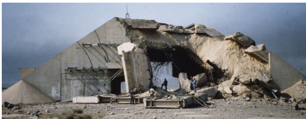
Figure 7: Iraqi Hardened Aircraft Shelter destroyed by coalition bombs during the Gulf War. 35
