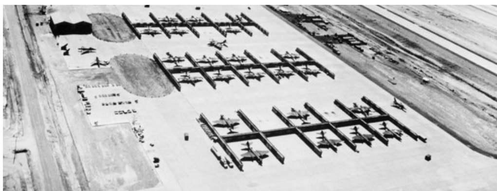
Figure 3: RAAF Canberra bombers in revetments at Phan Rang, South Vietnam. 16 Revetments provide protection from sides and rear, reducing damage from adjacent attacks.
