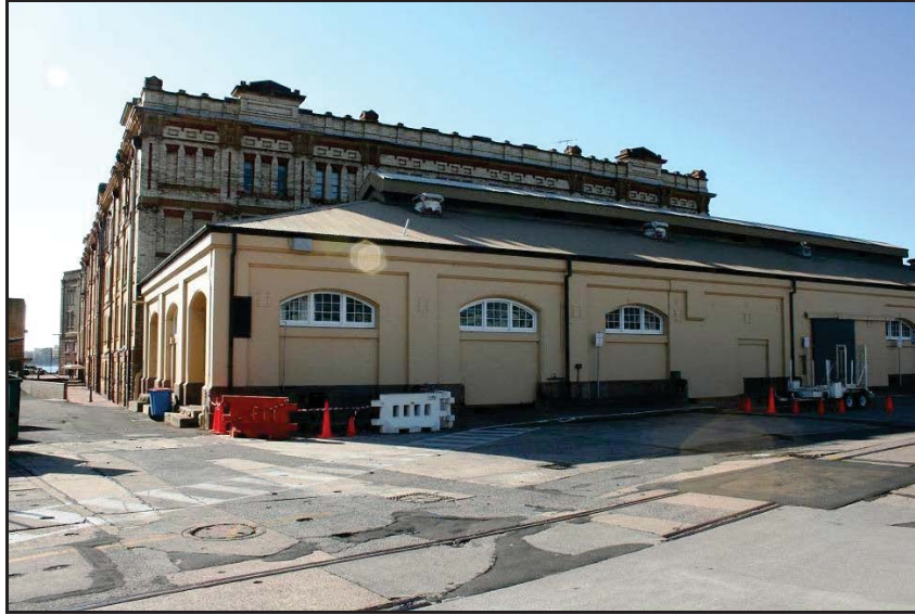
Figure 44 - View from the Cruiser Wharf of Building 89/90 (rear)
