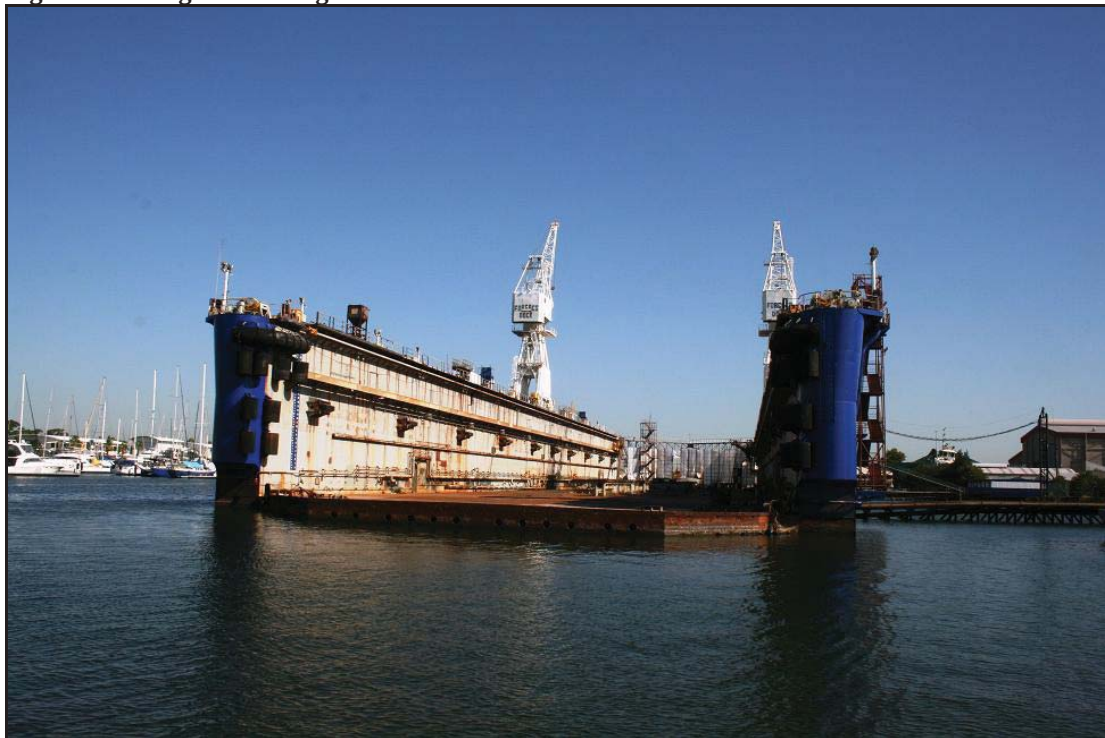
Figure 92 - Forgacs Floating Dock - Port of Newcastle
