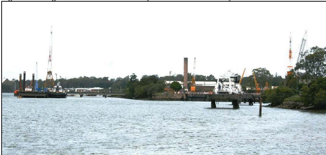
Figure 26 - Forgacs Cairncross Dock Facility - River View from Navy Wharf
