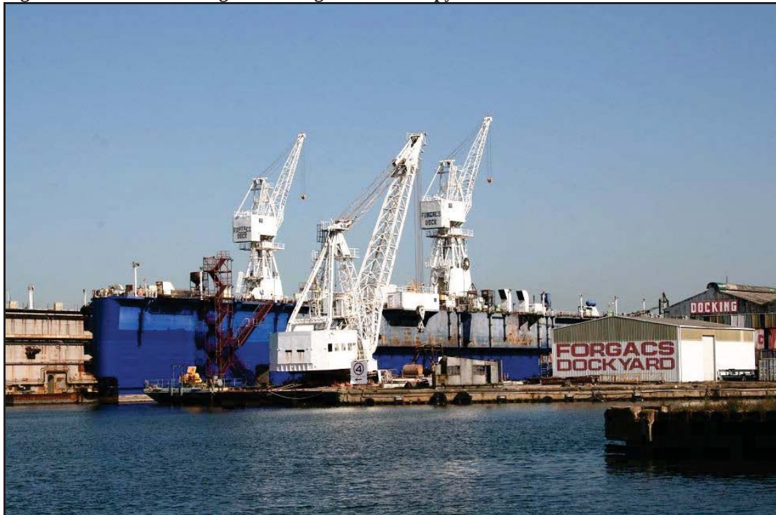
Figure 39 - Newcastle - Forgacs Floating Dock and Shipyard
