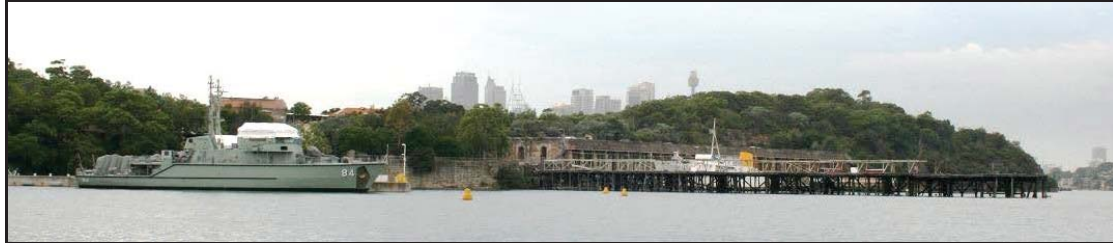
Figure 52 - East Wharf HMAS Waterhen with Coal Loader Wharf
