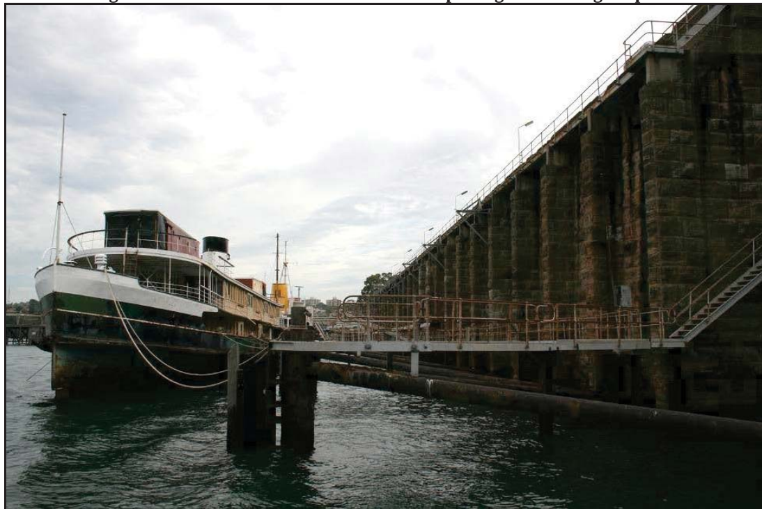
Figure 58 - Site of a Potential FSM Wharf replacing the Existing Dolphins
