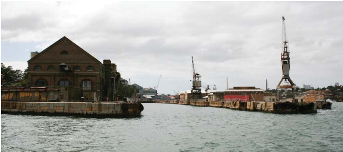
Figure 66 - Entrance to Sutherland Dock
