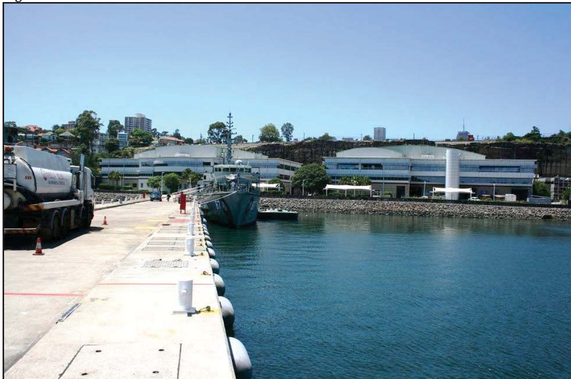
Figure 50 - HMAS Waterhen & Northern Wharf
