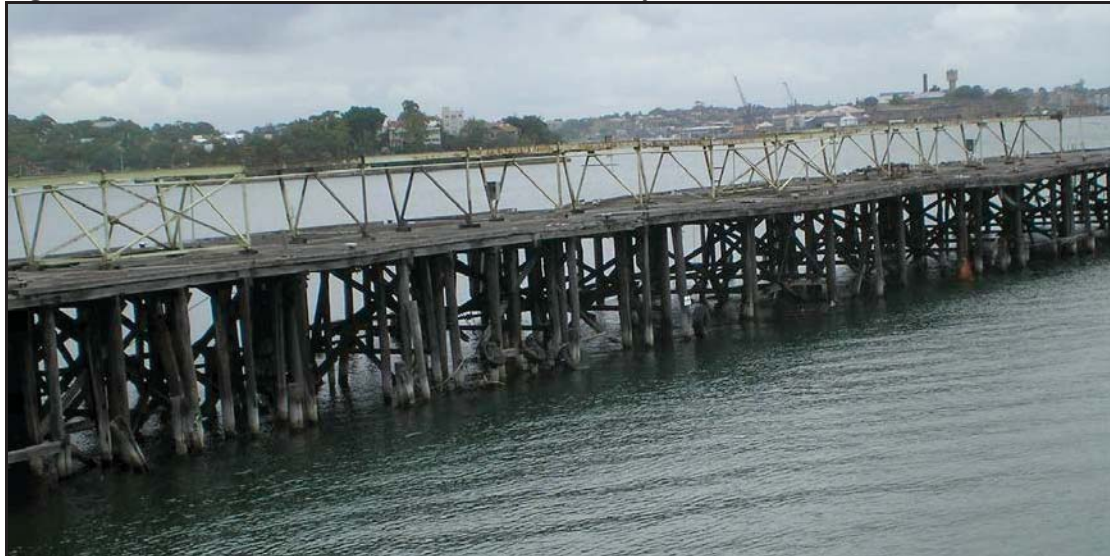
Figure 56 - Derelict Coal Loader Wharf - Balls Head Bay 258
