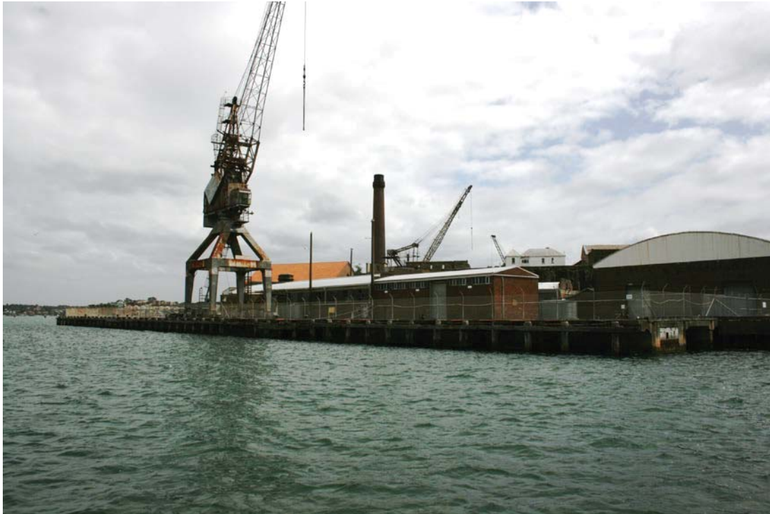
Figure 65 - South West Wharf Cockatoo Island
