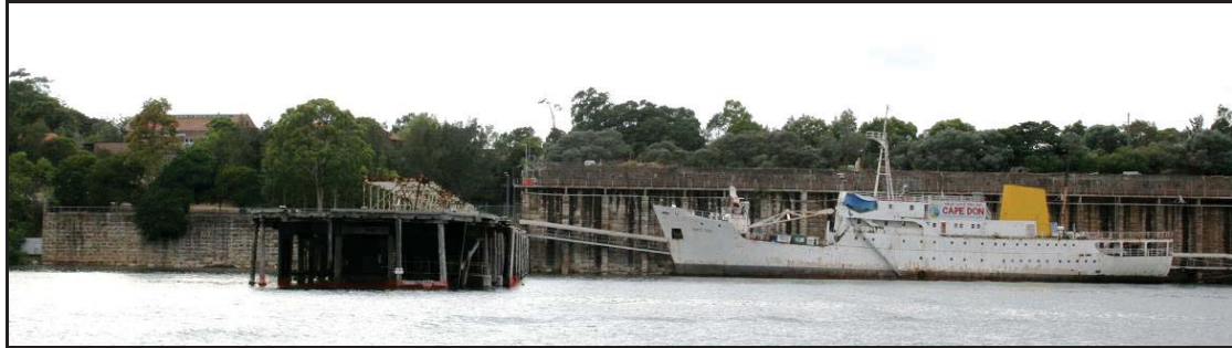
Figure 54 - Coal Loader - Ship Berthed at "NSW Maritime" owned Dolphins
