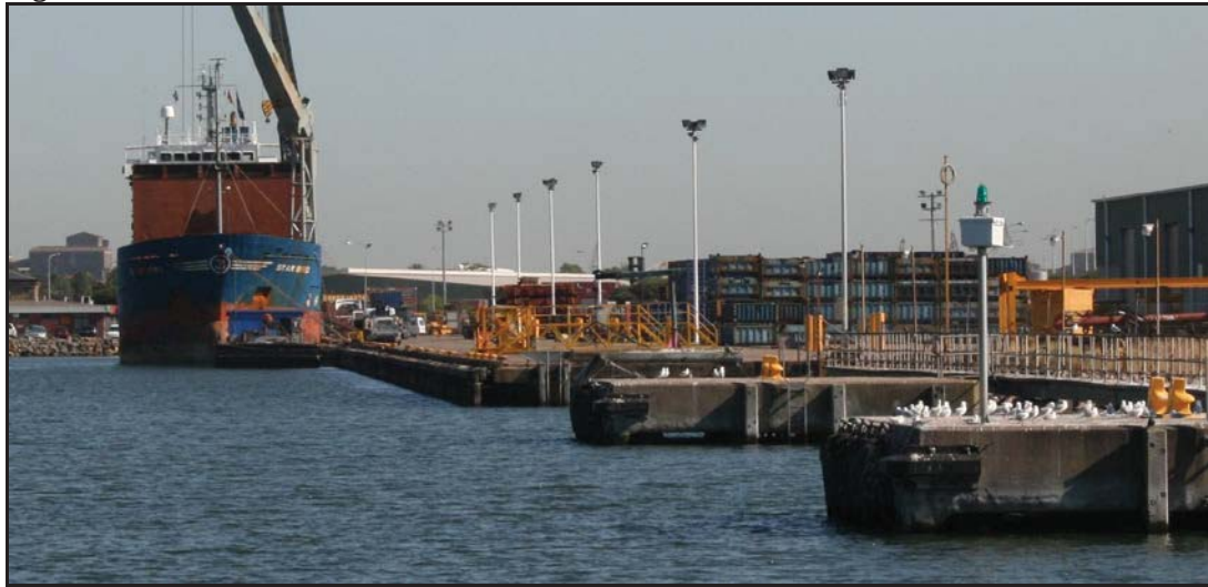
Figure 10 - Port of Newcastle Eastern Basin Wharf
