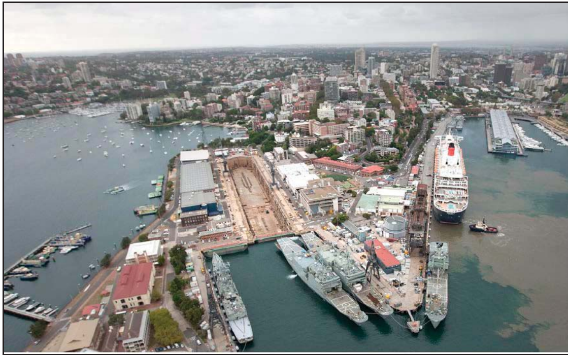
Figure 13 - Captain Cook Graving Dock - Sydney 96
