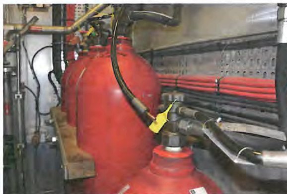
Figure 16: The pivotal hose detached from the fourth CO2 bottle.
