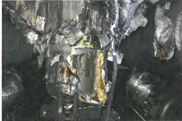
Figure 10: Damage lagging on the top of the king post.
