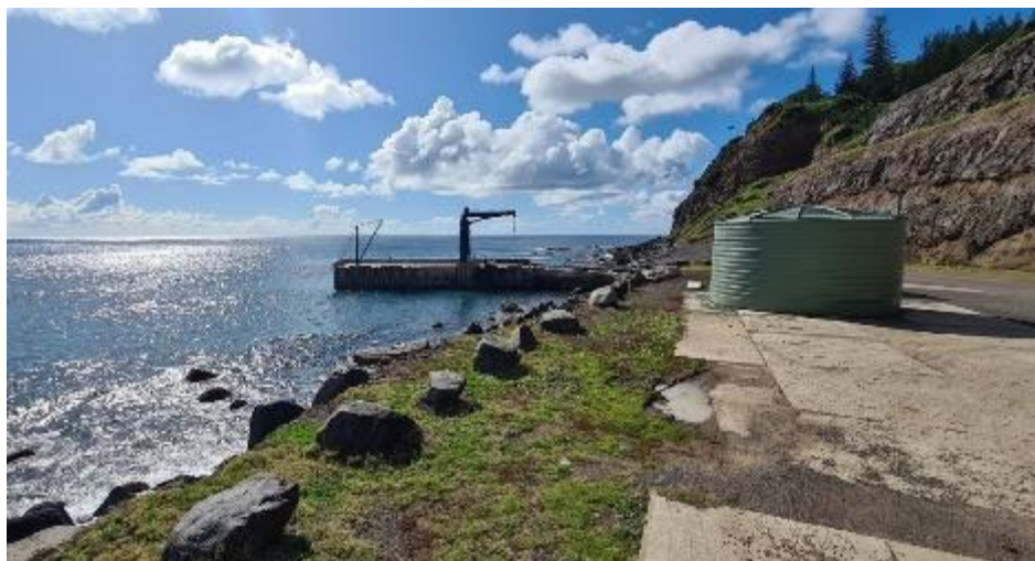
Figure 11: Cascade Pier Ground
