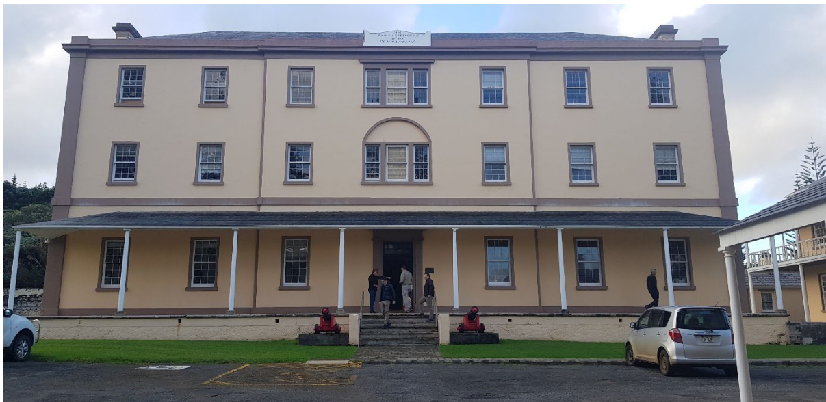
Fig 4: Shows the Norfolk Island Council offices within the 1836 Commandant's Building
