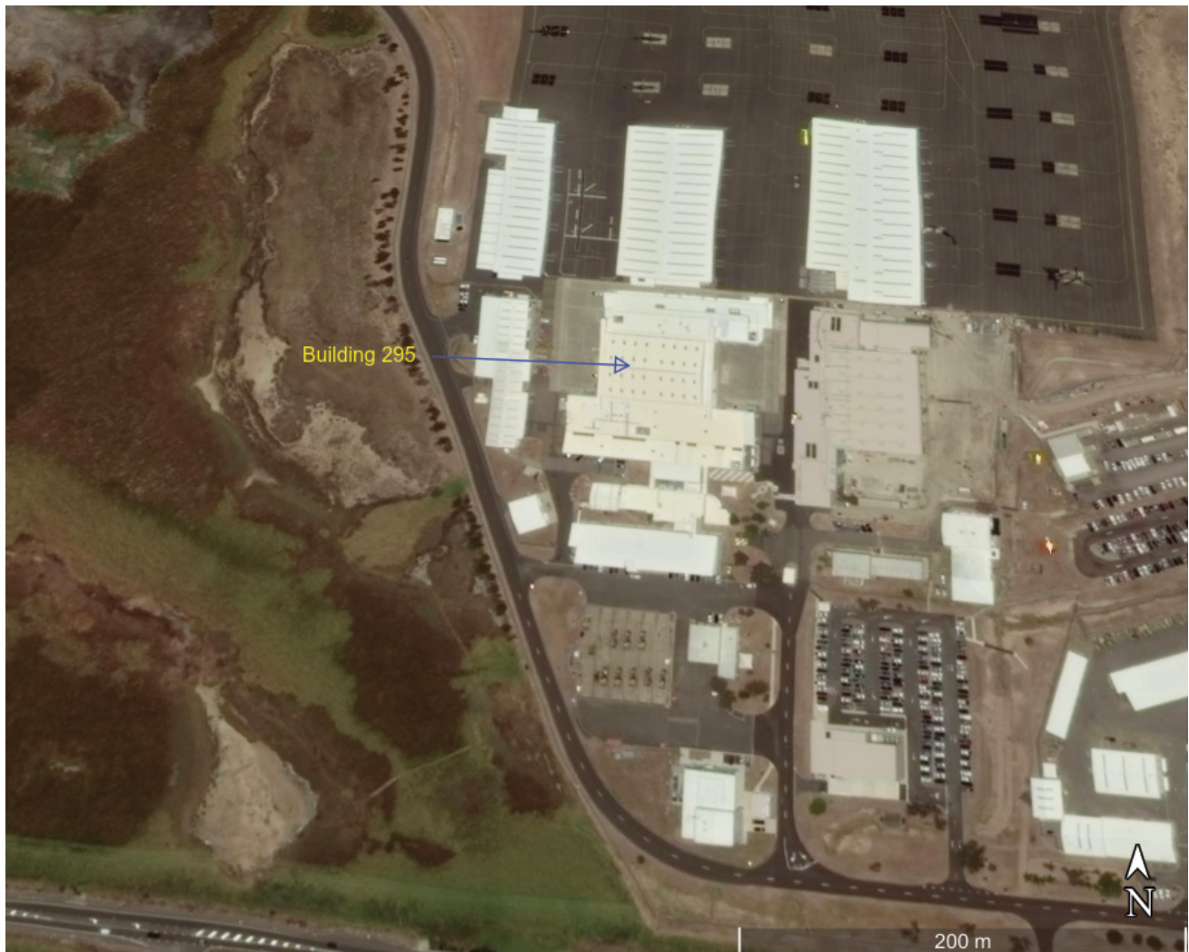
Figure 3.12 Building 295 (aerial view)
