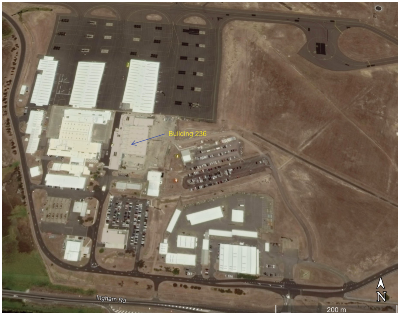
Figure 3.11 Building 236 (aerial view)
