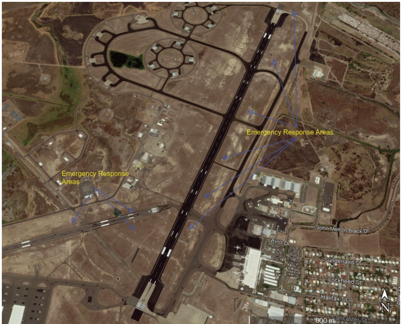
Figure 3.8 Emergency response area potentially impacted (aerial view)
