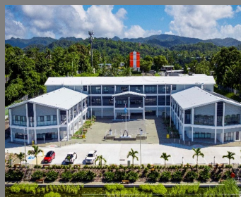
Maritime Essential Services Centre Fiji $100m
