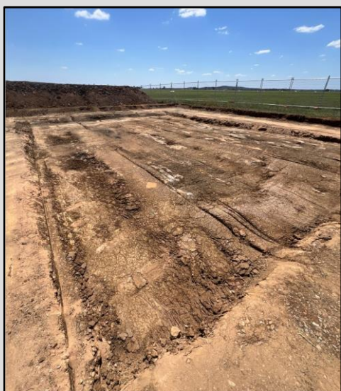
Excavation at the Former fuel compound.
