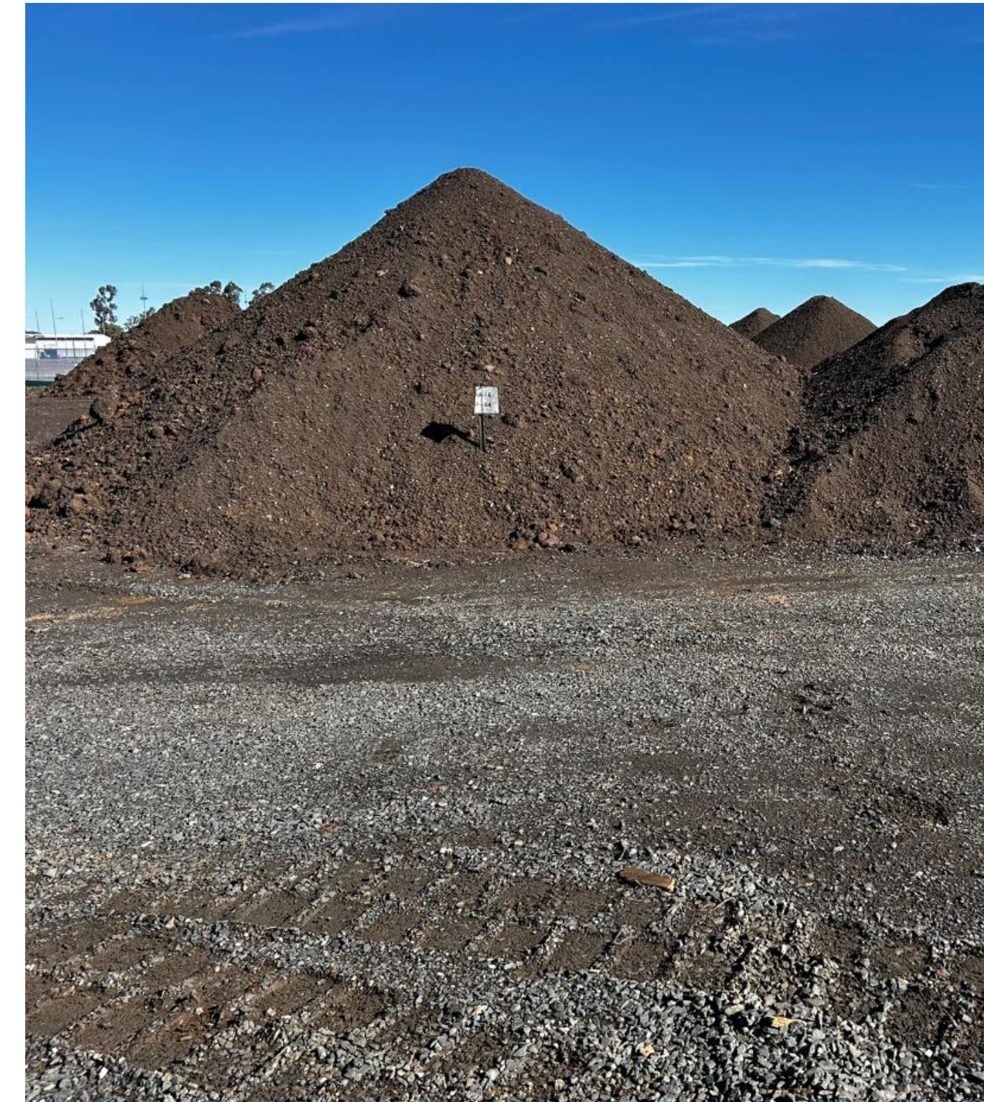
Soil stabilisation with powdered activated carbon on the Defence Estate, July 2025.
