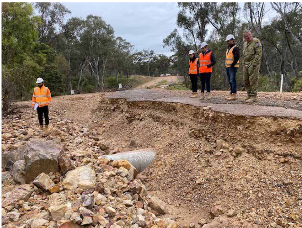
Photo: Flooding at the Puckapunyal Military Area caused damage to roads, culverts and bridges in during the October 2022 Victorian floods. Repairs costing approximately $2.5 million.
