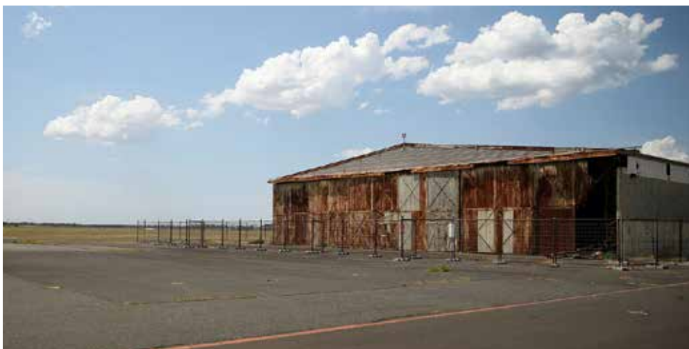
Photo: The Bellman Hangars at RAAF Williams—Point Cook, Victoria, are in an advanced state of disrepair and have been fenced off for safety reasons. The heritage value attributed to the hangars has seen them retained, but not restored. The corrosion of the building materials is evident in the picture and presents a significant health and safety risk.
