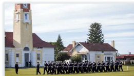
Heritage Building Works
