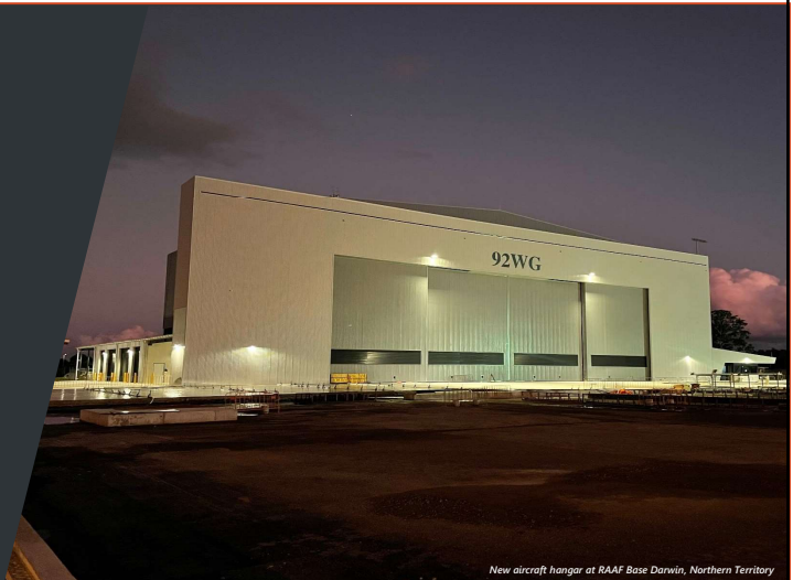
New aircraft hangar at RAAF Base Darwin, Northern Territory
