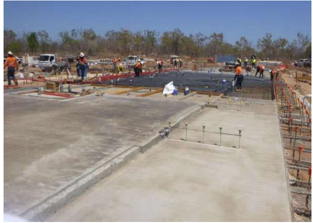
Construction of new living-in accommodation at RAAF Base Tindal NT
