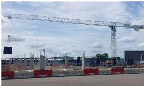
Construction to support new Apache Helicopter Capability at RAAF Base Townsville
