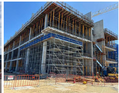
Construction under the Submarine Rotational Force West Project at HMAS Stirling
