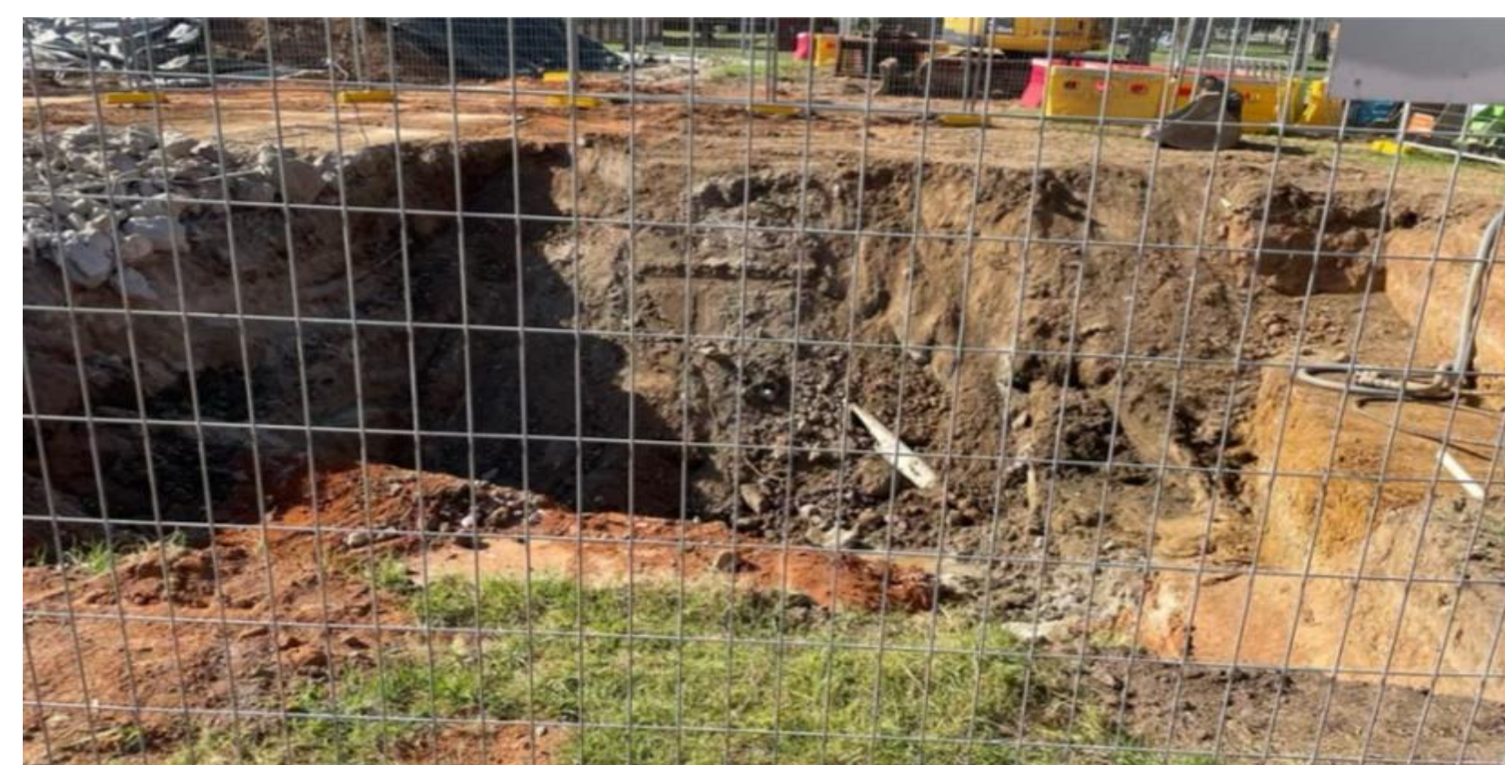
Removal of wastewater collection tanks
