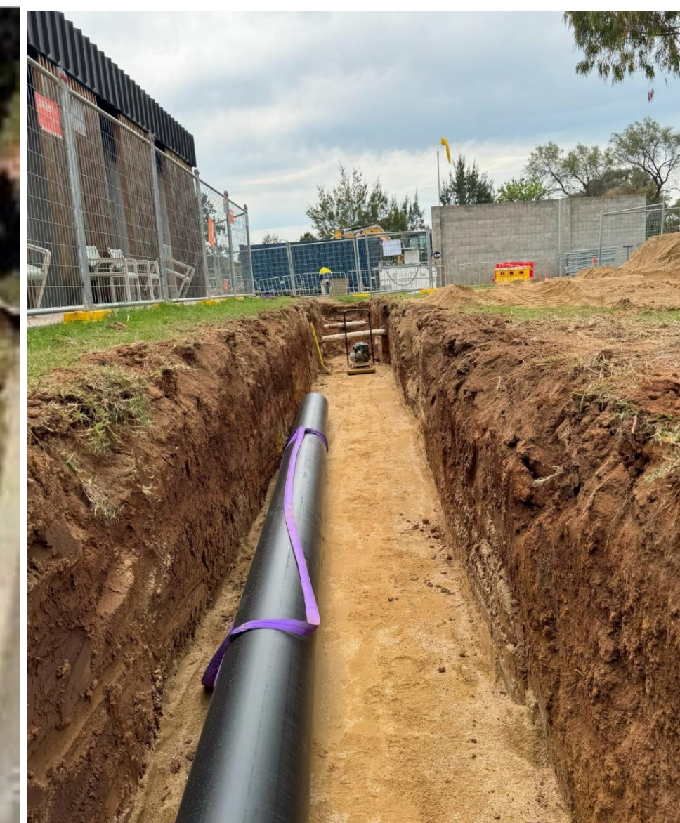
Replacement of stormwater pipes
