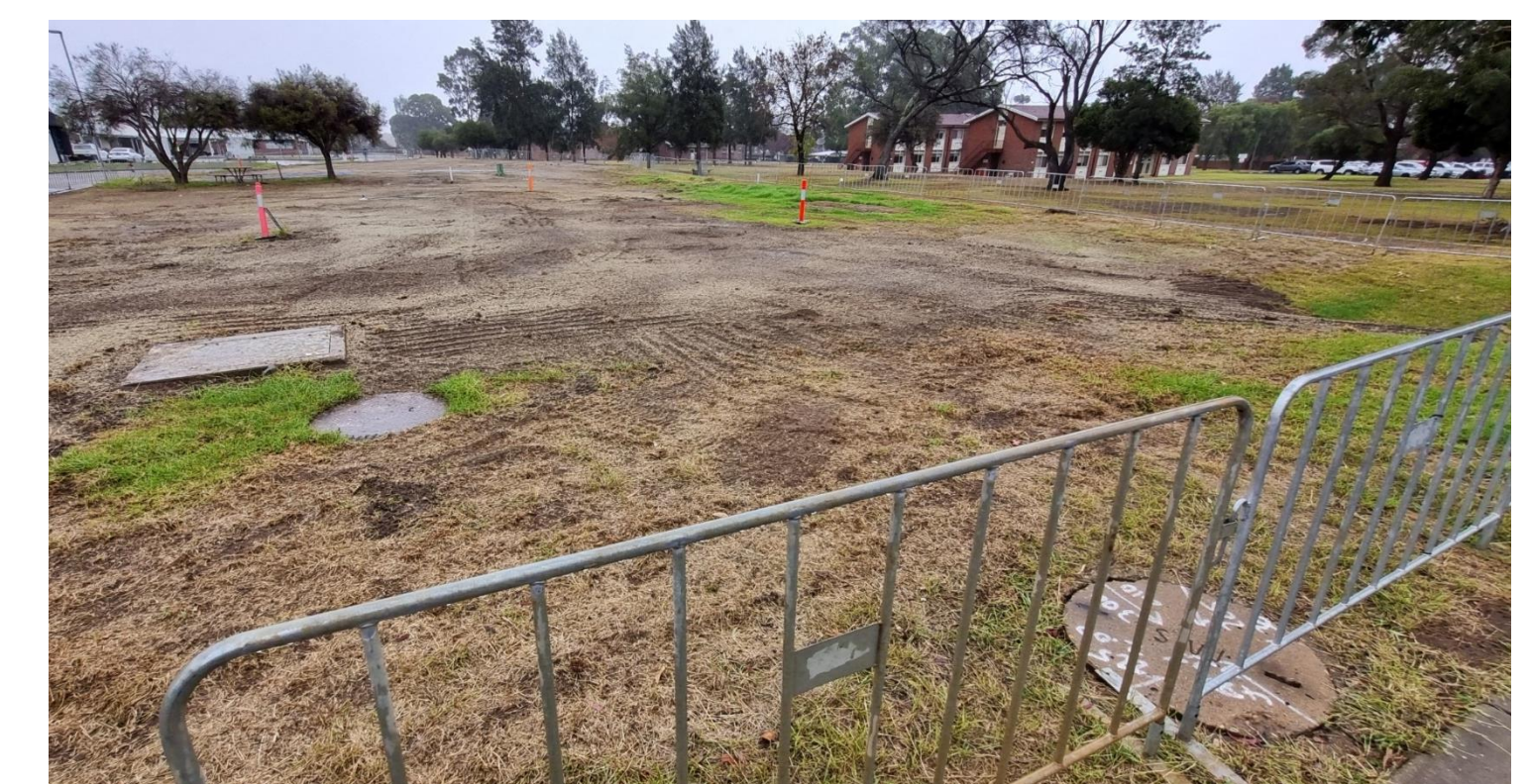
Completion of remediation works
