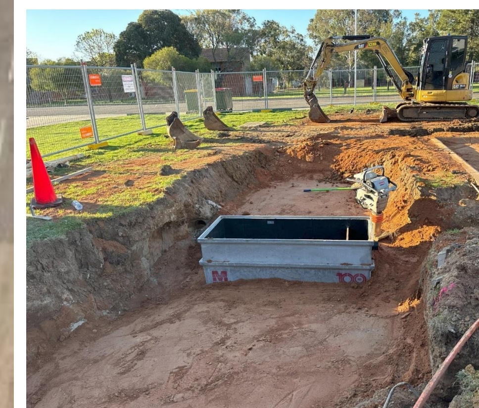
Replacement of oil/water separator
