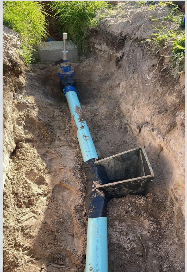
Pictured: Water mains being installed in South Bullsbrook.
