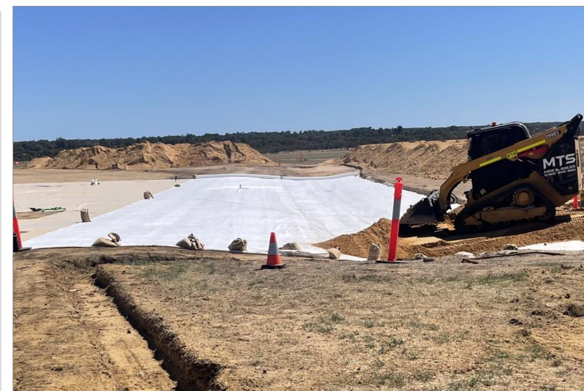
Placing the liner over contaminated soil in March 2025.
