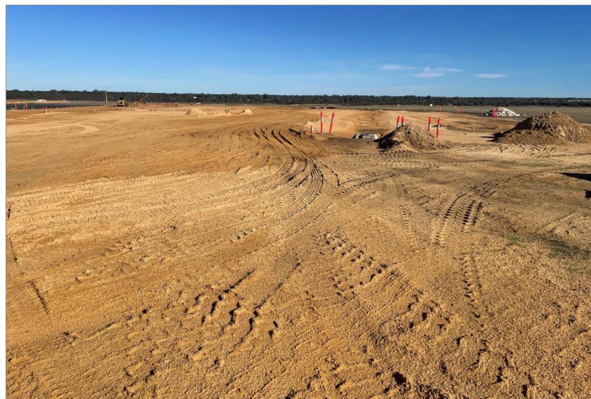
Placing clean sand over the liner in April 2025.
