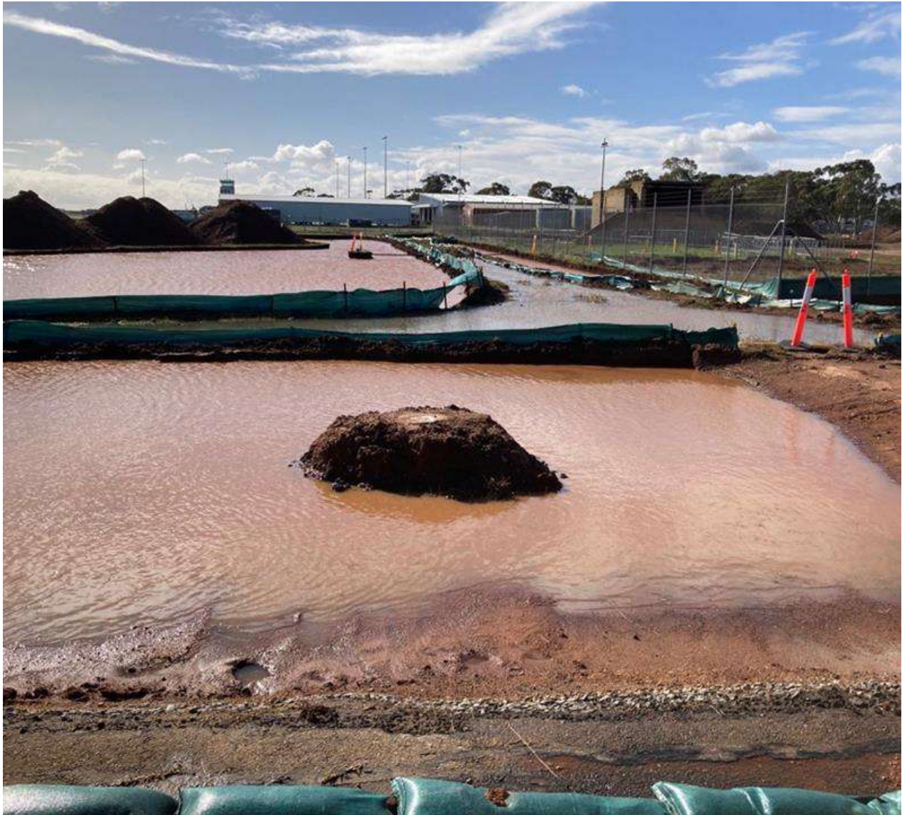
Figure 1 P9 excavation 6 June 2022
