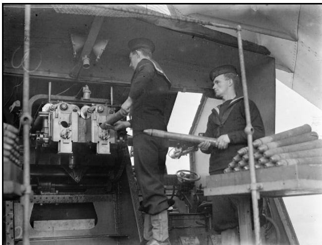
Figure 3 – 6 pr loading drill on British destroyer HMS Mackay (IWM photograph A 20313)
