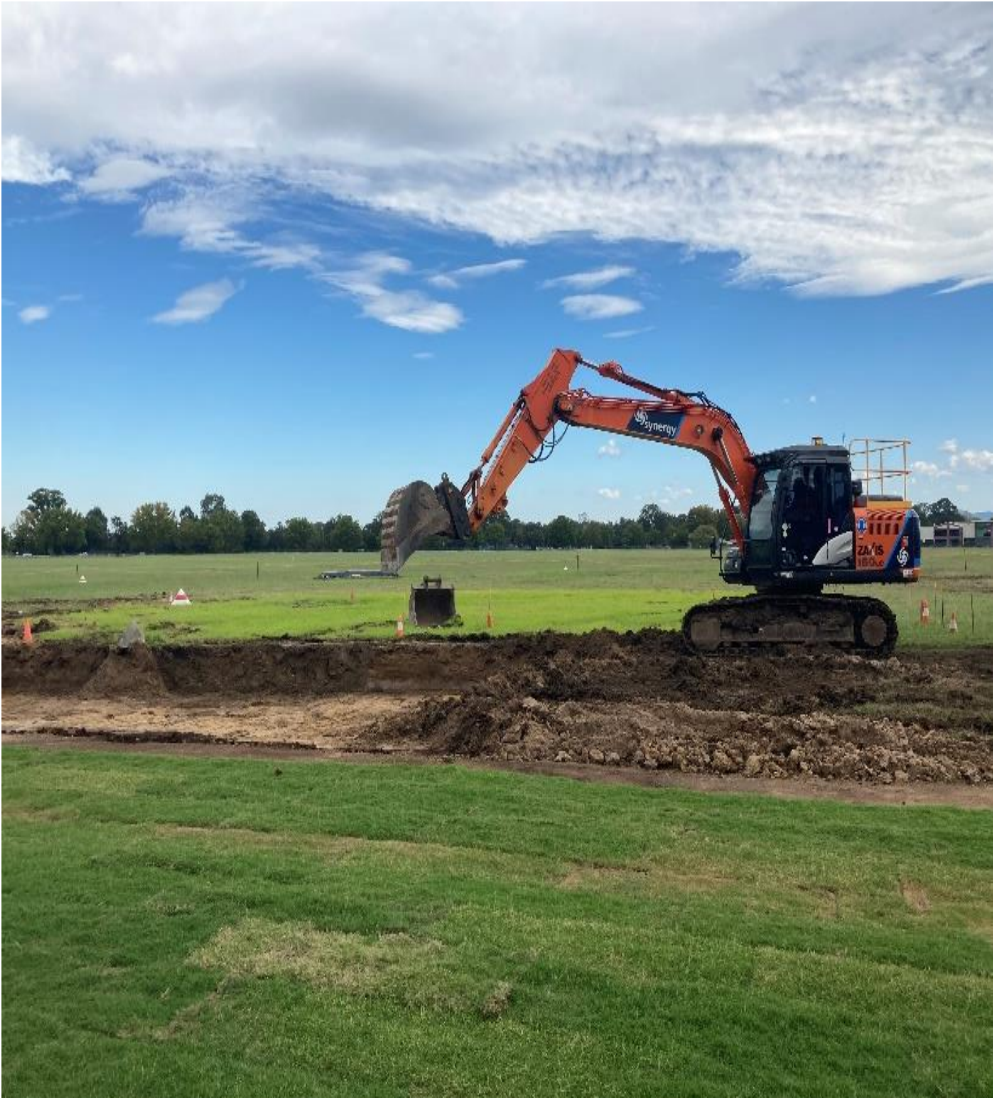
Soil stabilisation underway on the Defence Estate
