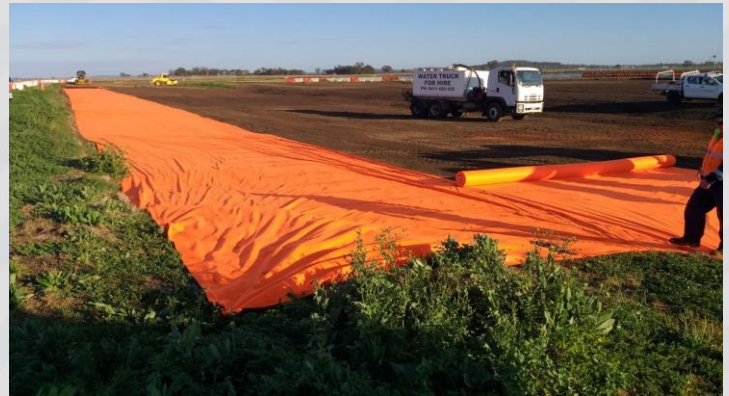
Soil remediation - installation of geo-fabric marker layer
