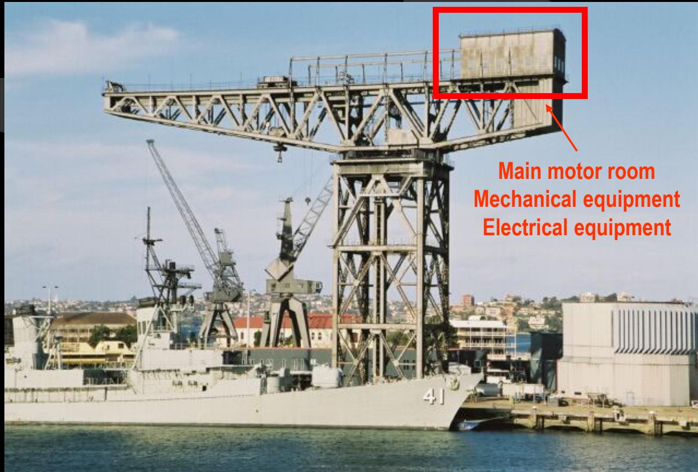
Hammerhead Crane at Garden Island Naval Base - Sydney
