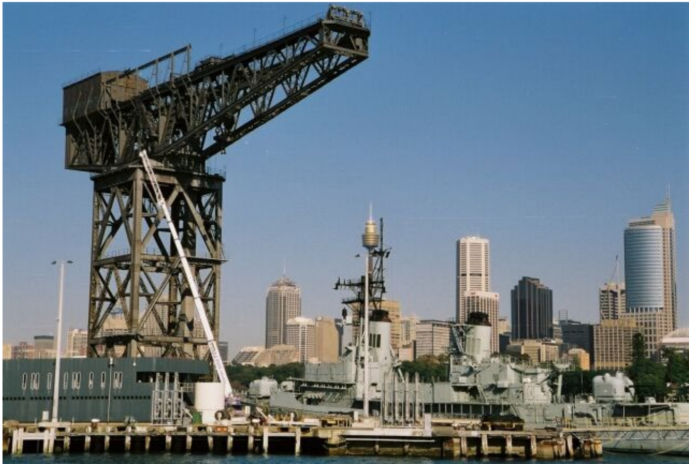
Figure 1: The Hammerhead Crane and Sydney CBD, 2003 (Source: Robert Bird & Partners, 2003, Condition Study of the Hammerhead Crane)
