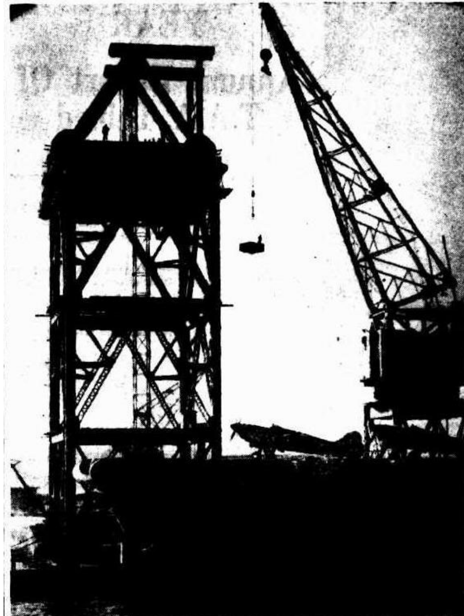
Size of the 250-ton-capacity crane which is being built at Captain Cook Dock, Garden Island, is illustrated in this picture. In the foreground is the bow of the aircraft-carrier Sydney, with the crane towering in the background. Total weight of the structural steel in the crane is 1,400 tons.
