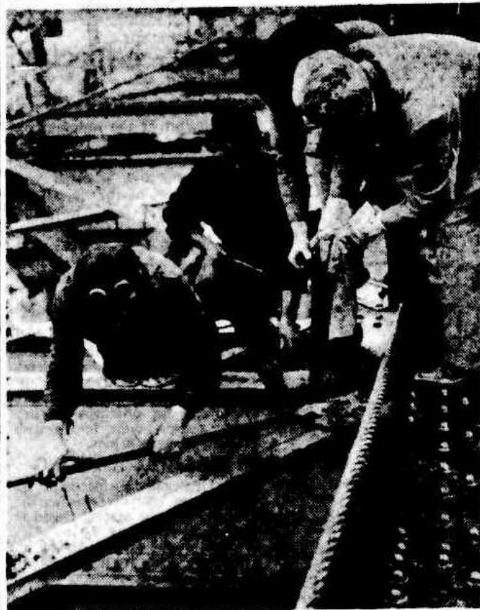
The former Director of Works and Housing, Mr. M. W. Mahaffey, drives the last rivet into the framework of the new Captain Cook dock crane at Garden Island yesterday. The picture was taken 254 feet above the ground.
