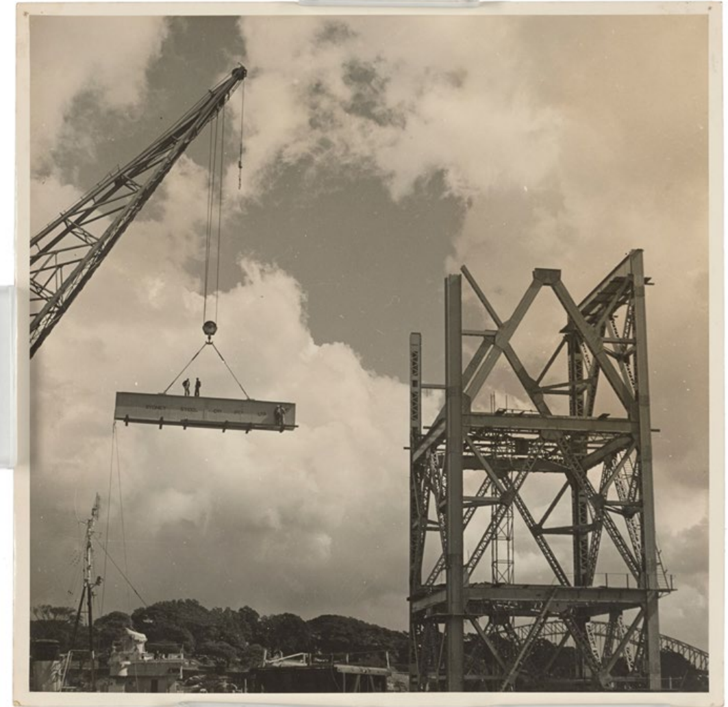
Figure 17: Photograph of the Hammerhead (Giant Titan) crane (Source: Sydney Steel Company Pty Ltd, Photographed by Colin Stuart, 1948 – 1951 Item No. 2014/39/1-35)
