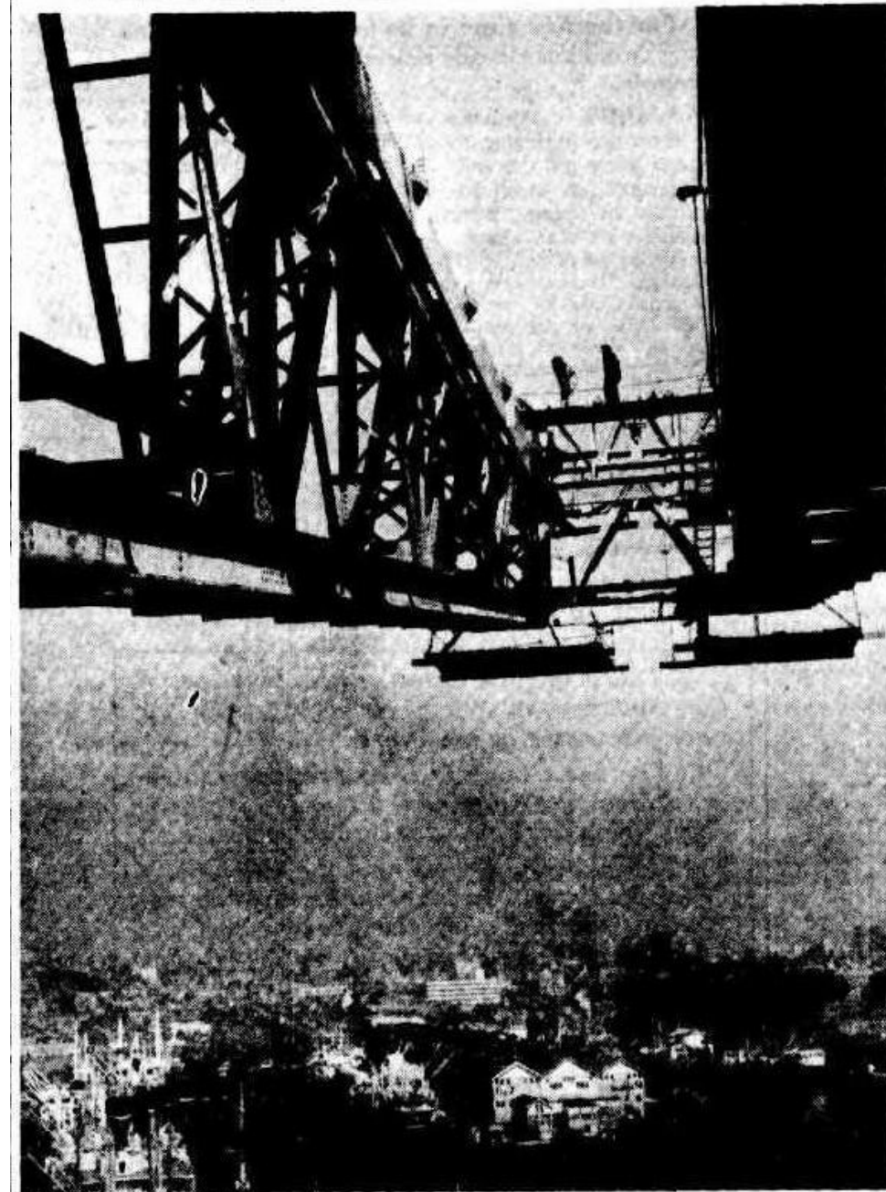
Shipping and buildings at Woolloomooloo are dwarfed by the nose piece of the 270-foot jib of the cantilever crane being constructed at Captain Cook Graving Dock. The crane will have a lift of 250 tons.
