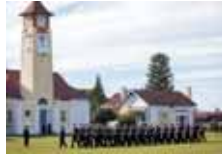
Heritage Building Works
