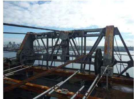
Jib Tip Cable Anchorage Frame
