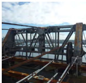
Jib Tip Cable Anchorage Frame (Source: GML)
