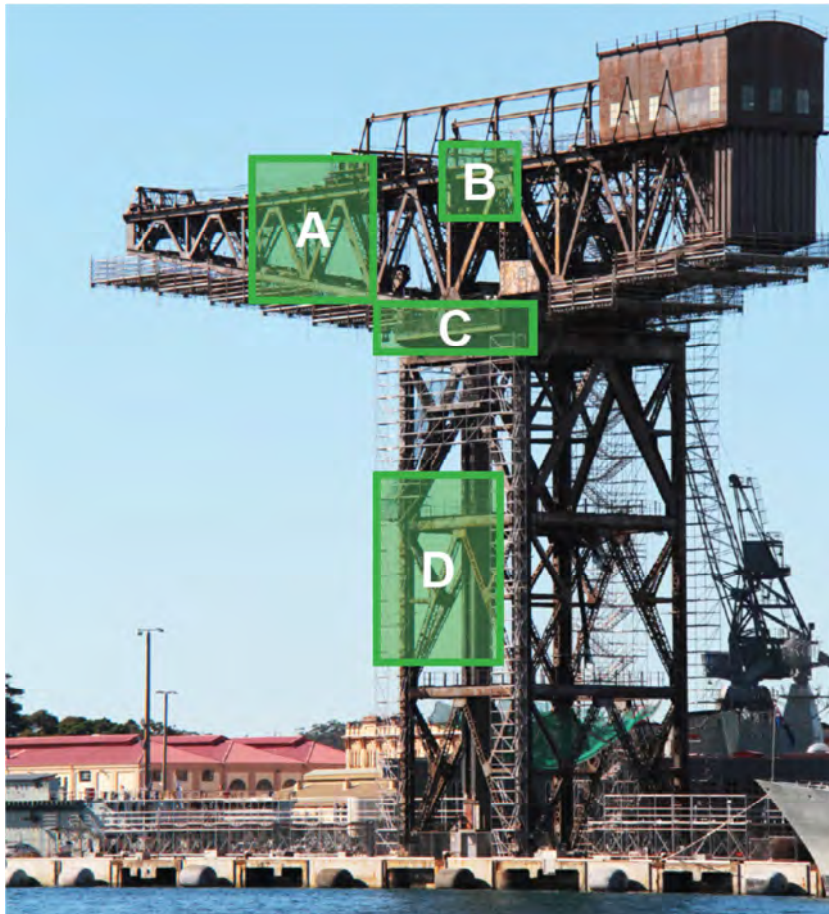
Figure 3.1 Indication of where components A, B, C and D would be sourced from the Hammerhead Crane. (Source: GML 2013)
