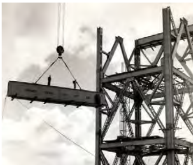
Figure 2.23 Erection of the second girder c1949. (Source: Sydney Steel Archives Warwick Stuart)
