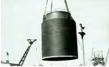
Figure 2.21 Foundation cylinders being installed. (Source: Naval Historical Society)
