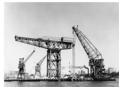
Figure 2.27 1965 view of the Hammerhead Crane and the floating Titan Crane. (Source: Naval Historical Society)
