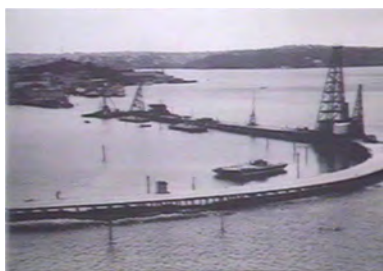
Figure 2.7 1941 image of Captain Cook Graving Dock under construction. (Source: SLNSW)
