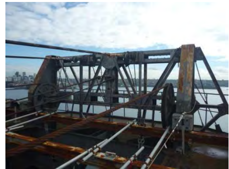
Jib Tip Cable Anchorage Frame
