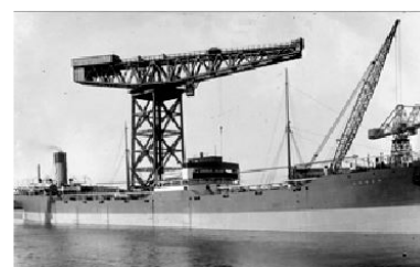
Figure 2.12 Titan Hammerhead Crane in Clydebank, UK built in 1907. (Source: Flickr)
