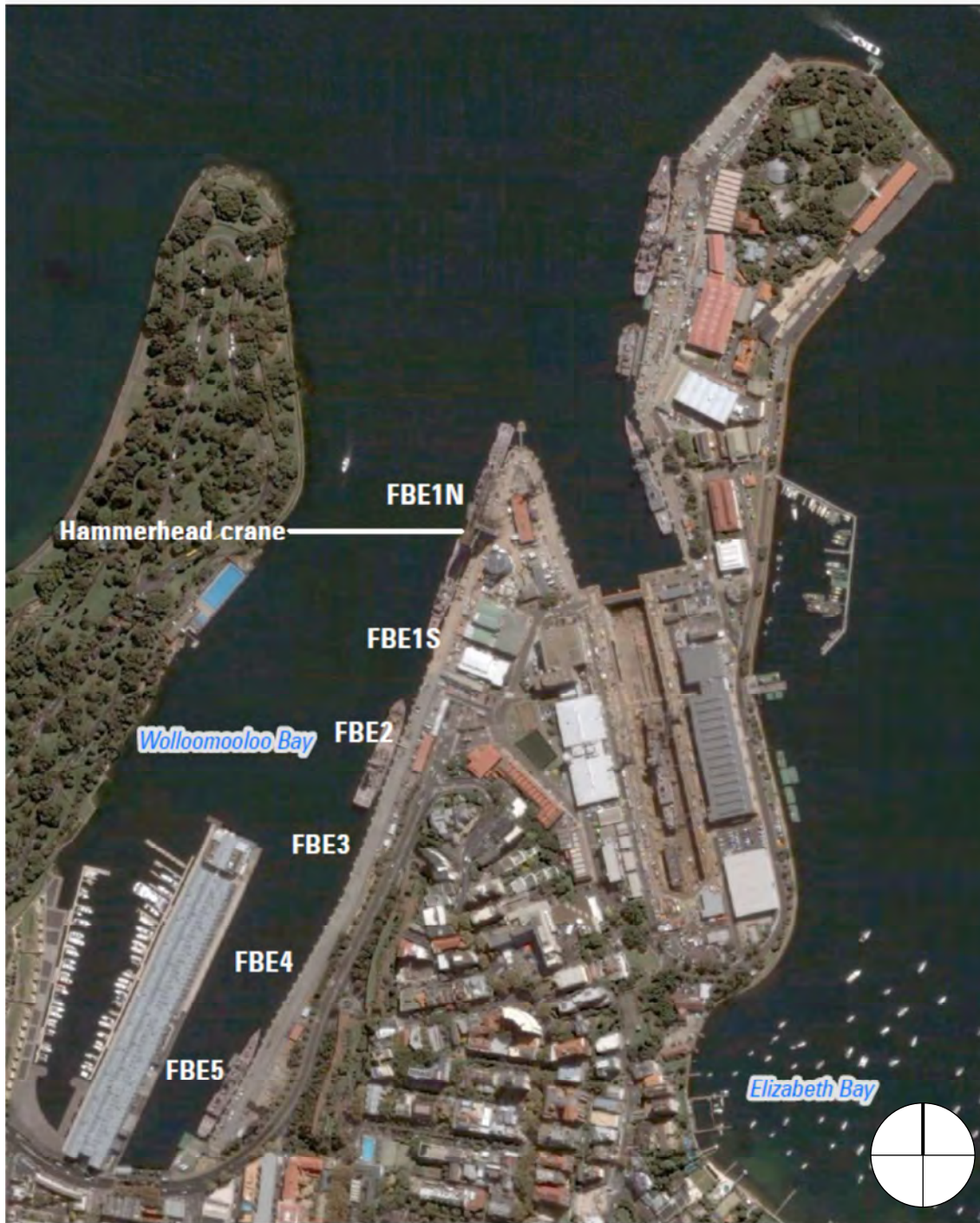
Figure 1.2 Garden Island aerial with the Hammerhead Crane (Defence Asset 76) at FBE1N and associated wharves. (Source: Parsons Brinkerhoff 2012)
