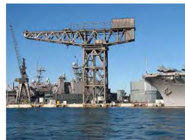
Figure 2.10 Sydney's Hammerhead Crane. (Source: Dr Iain Stuart)
