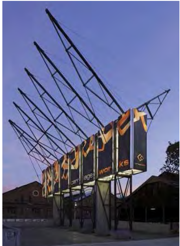
Re-use of the former 1888 Carriage Workshops original trusses, as entry signage for the CarriageWorks Contemporary Arts Centre in Sydney.
