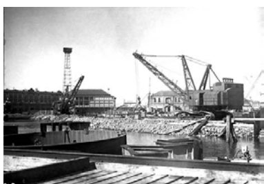
Figure 2.8 Captain Cook Graving Dock under construction. (Source: State Records 9856_a017_A017000063)
