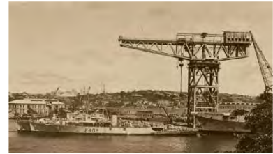
Figure 2.25 1950 view of the Hammerhead Crane. (Source: Dr Iain Stuart)
