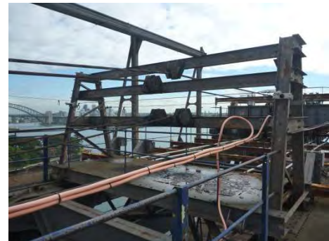
Mid Jib Cable Anchorage Frame
