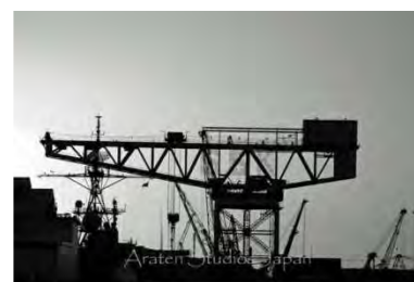
Figure 2.13 Sesbo Hammerhead Crane Japan, built in 1913 at Sasebo Naval Shipyard by Sir William Arrol and still standing. (Source: Araten Studios Japan)
