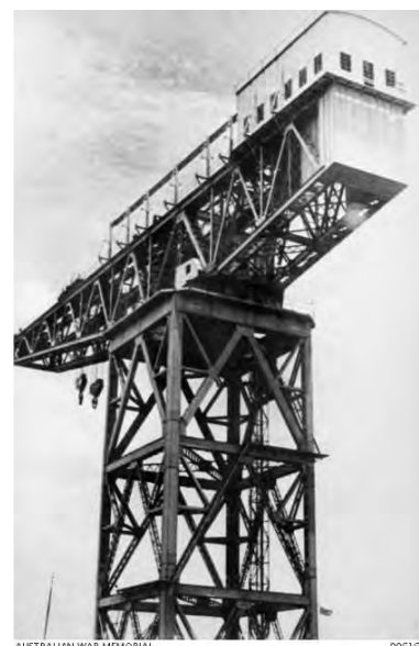
Figure 2.11 Singapore Naval Base Hammerhead Crane 1941–1943. (Source: Australian War Memorial)
