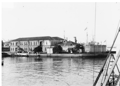
Figure 2.6 Garden Island just prior to the construction of the Captain Cook Graving Dock. (Source: State Records 9856_2017_2017000253)
