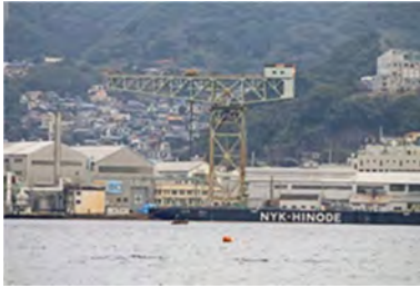
Figure 2.14 Nagasaki Hammerhead Crane, Japan. (Source: Dr Iain Stuart)
