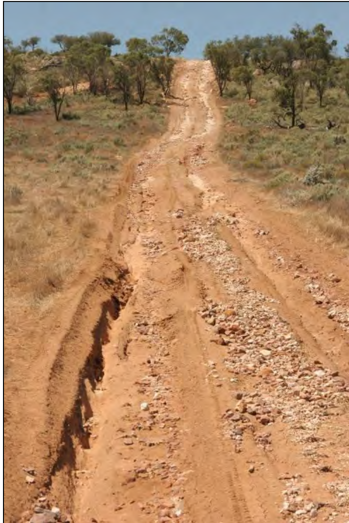
Figure 75. Erosion of track down the escarpment in sector T.
