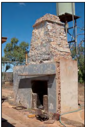
Plate 36 Stone fireplace/oven of second homestead
