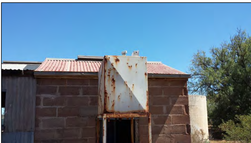
Plate 11: AST at the rear of the workshop
