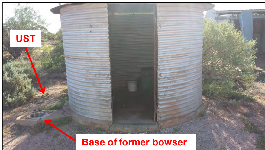
Plate 1: Oil and fuel storage shed near Main Homestead with adjacent UST and former bowser (approx. 100 m WSW of HS)
