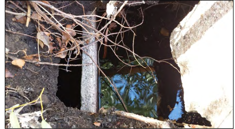
Plate 22: View inside interceptor pit
