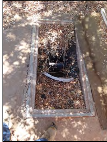
Plate 21: Interceptor pit adjacent to Middelback Homestead near main kitchen
