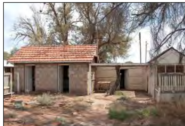
Plate 5 Storage shed, laundry and cool room
