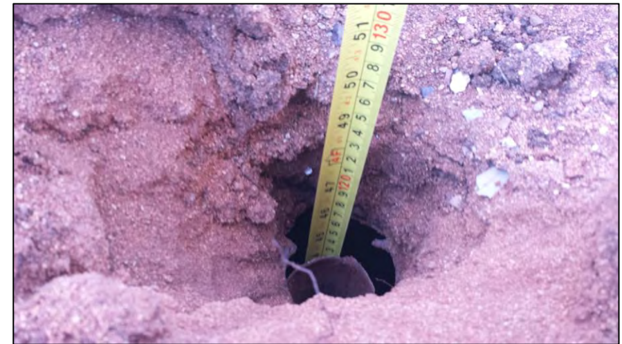
Plate 4: Internal depth of UST (approx. 1.2 m)
