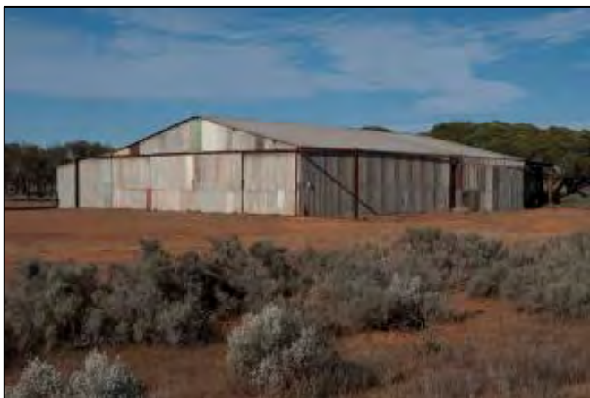
Plate 26 Overview of Whyalla Gliding Club Hangar
