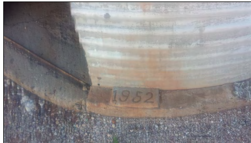
Plate 6: Concrete plaque on base of oil and fuel storage shed potentially indicating year of construction (1952)
