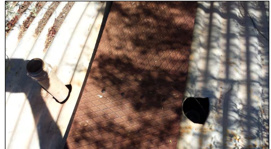
Plate 2: Top of UST showing fill point and dip point
