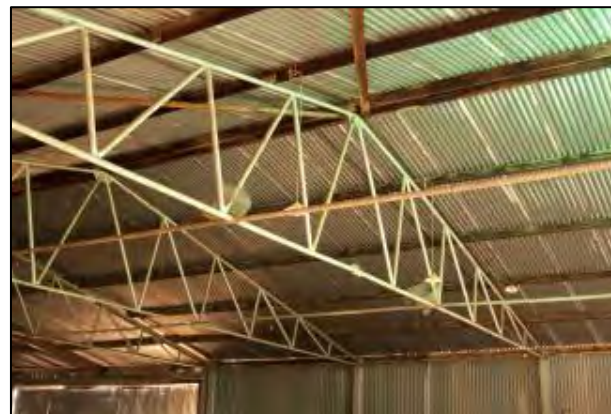
Plate 29 Whyalla Gliding Club Hangar (construction detail)
