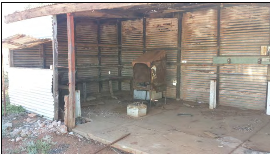
Plate 15: Former blacksmith workshop (approx. 280 m ESE from Original Homestead)
