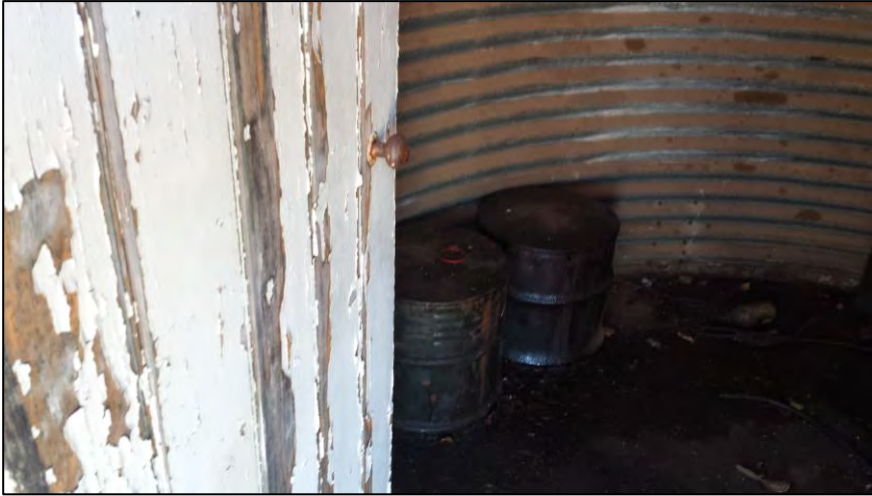
Plate 9: Oil / fuel storage drums inside oil and fuel storage shed
