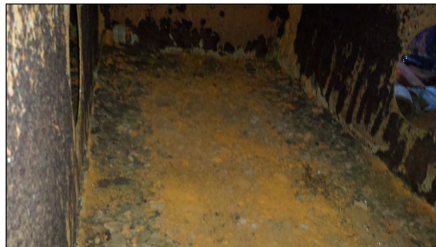
Plate 20: View inside storage tank of unknown use
