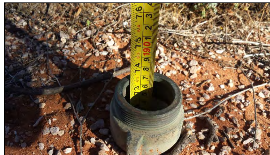
Plate 4: Internal depth of UST (approx. 1.8 m)
