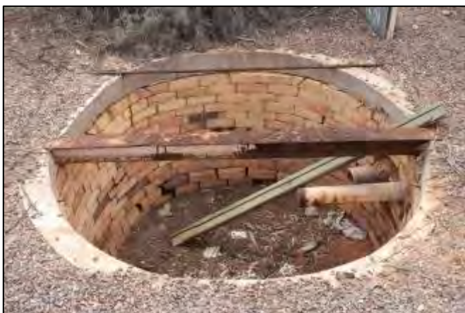
Plate 4 Brick lined septic well
