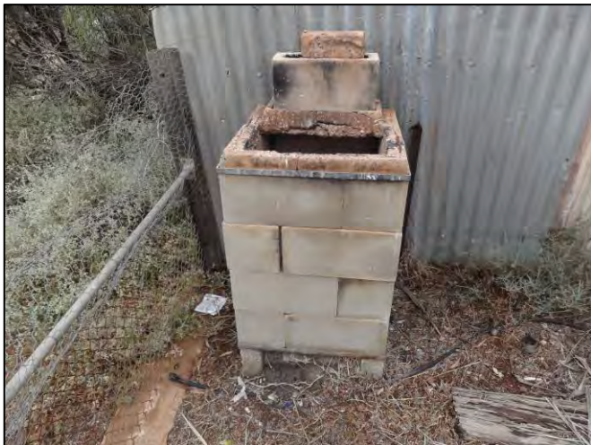
Plate 9: Small domestic incinerator near Manager's House
