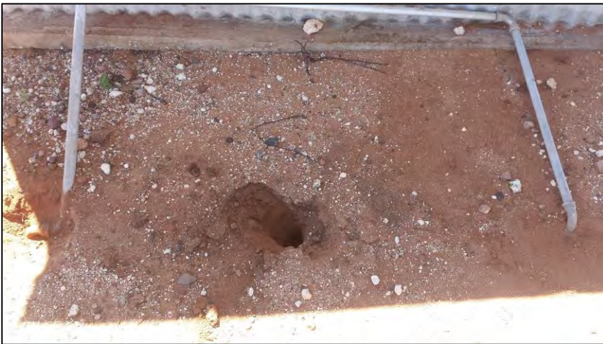
Plate 3: UST fill point, breather pipe line and fuel transmission line
