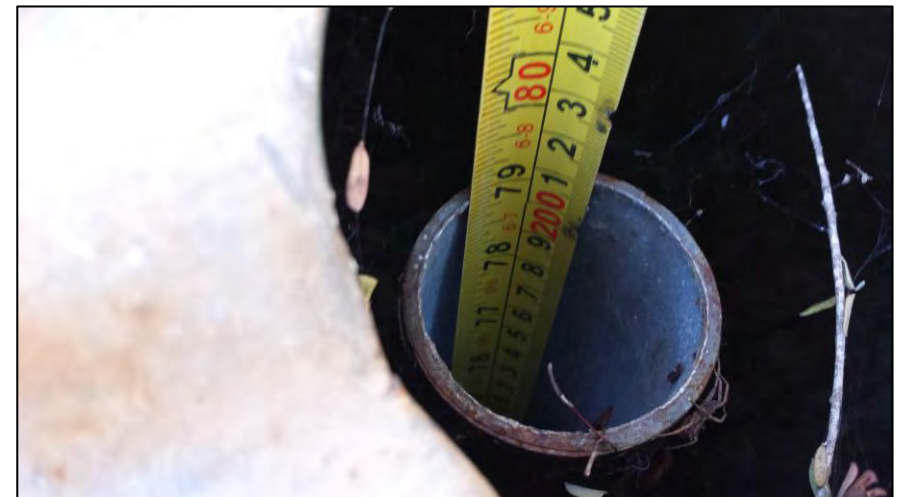
Plate 4: Internal depth of UST (approx. 2 m)
