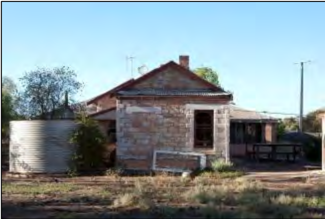
Plate 14 Extension at northern end of main homestead
