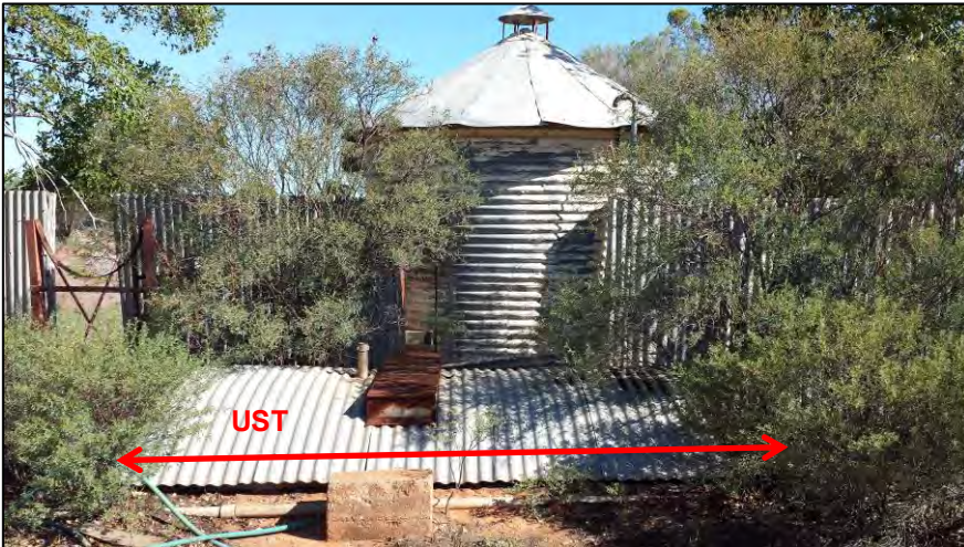
Plate 1: UST at rear of oil and fuel storage shed near original Homestead
