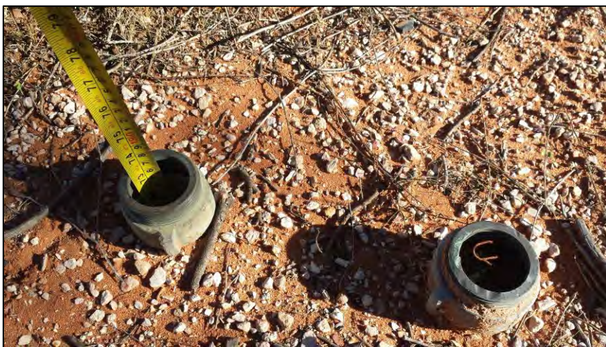
Plate 3: UST fill point and dip point
