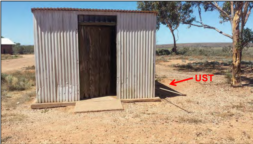
Plate 1: Oil and fuel storage shed near Main Homestead with adjacent UST
