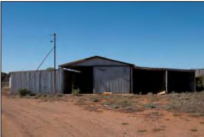
Plate 16 Workshop and vehicle storage sheds
