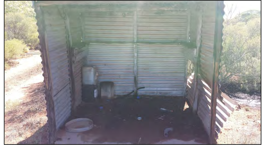
Plate 10: Second oil storage shed near vehicle service pit and waste oil soakage pit, near original Homestead
