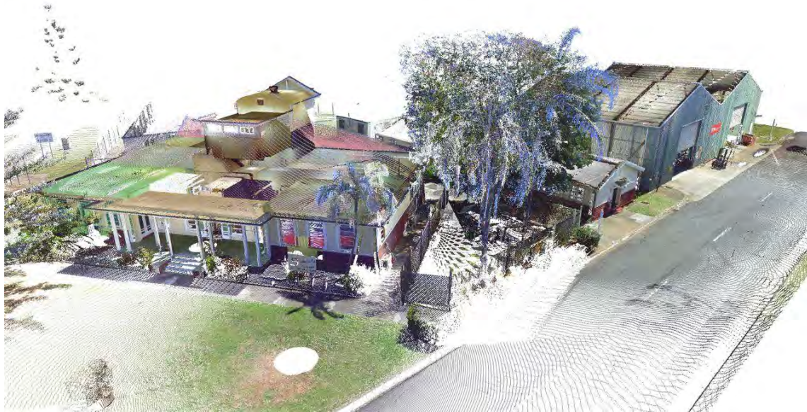
Figure 6 Image of 3D terrestrial scan of former Base Headquarters (RPS 2015)
