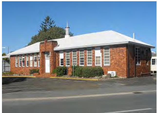
Plate 12 Hospital building (Amberley History n.d.:4)
