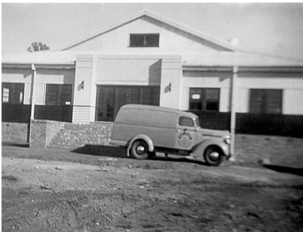
Plate 18 Astra Cinema under construction in 1941 (Amberley History n.d.:5)
