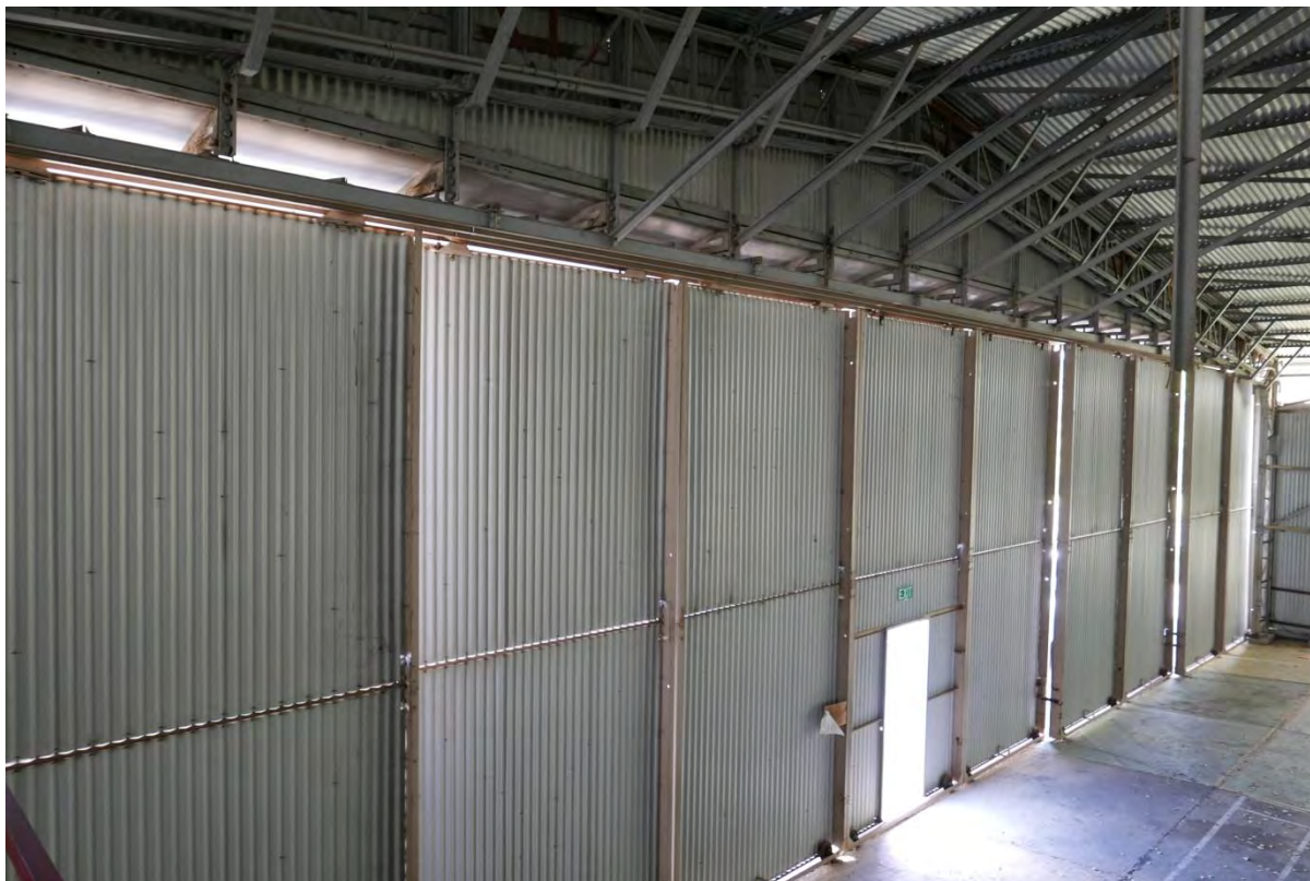
Plate 16 Hangar 261 – View of south doors from mezzanine - image 10654
