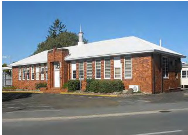
Plate 12 Hospital building (Amberley History n.d.:4)
