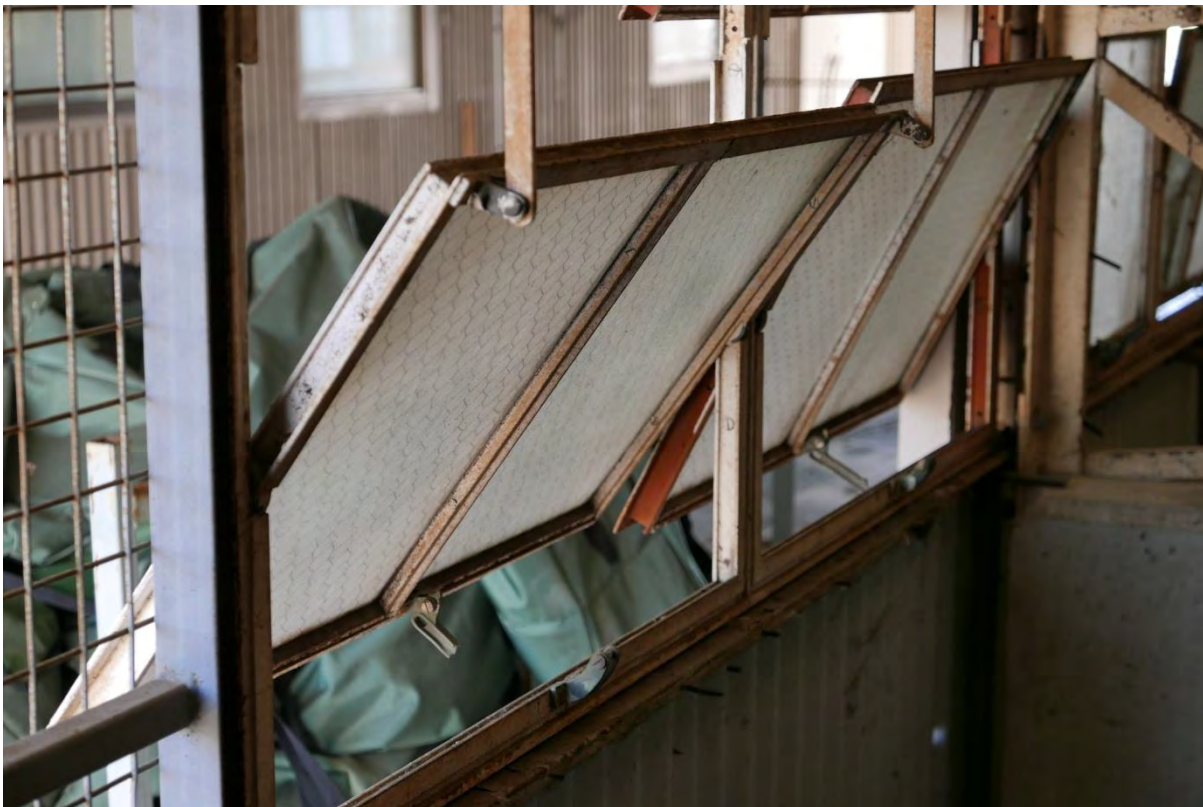
Plate 14 Hangar 257 – Steel framed windows in lower pane – image 10506
