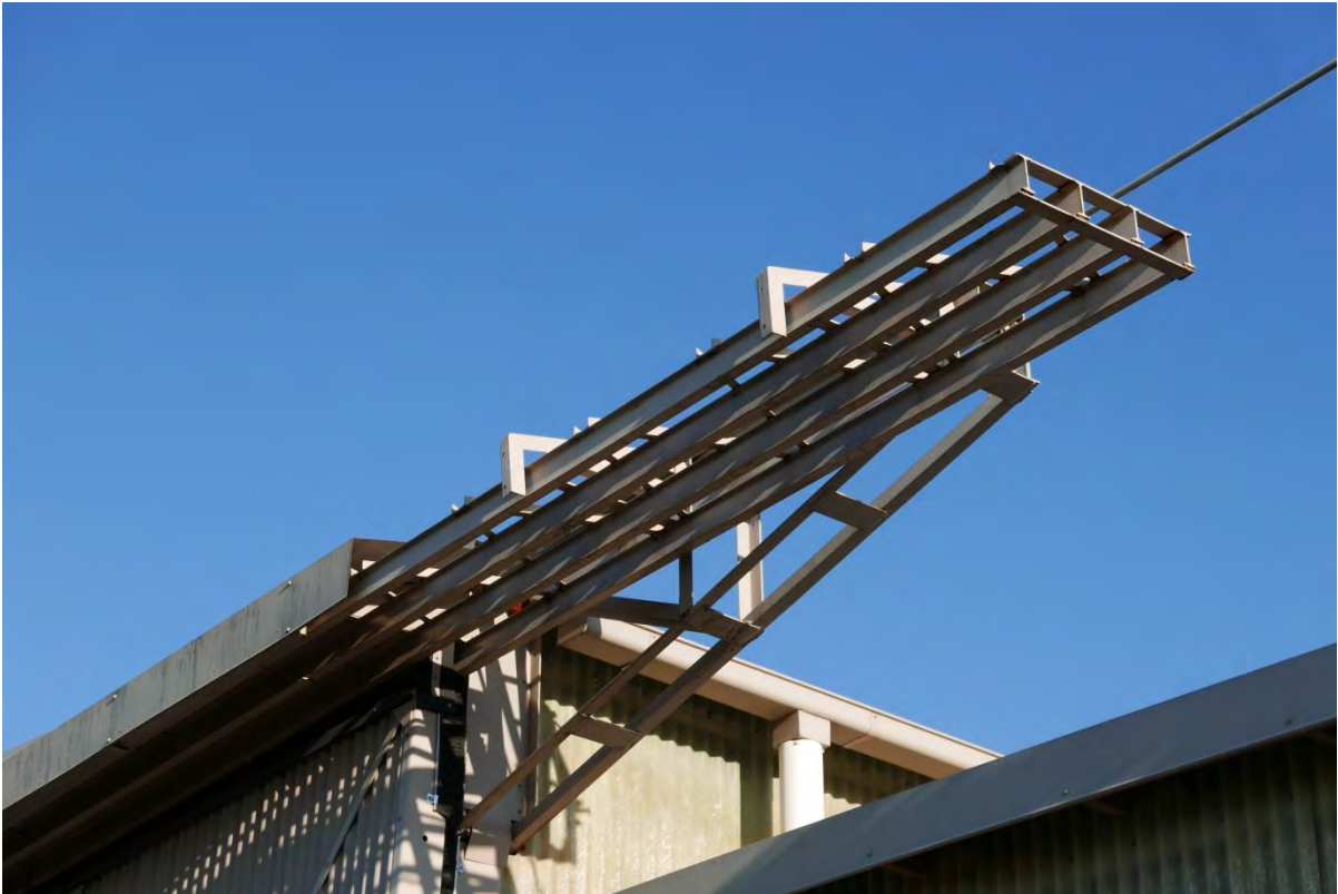
Plate 11 Hangar 258 door tracks – image 10313
