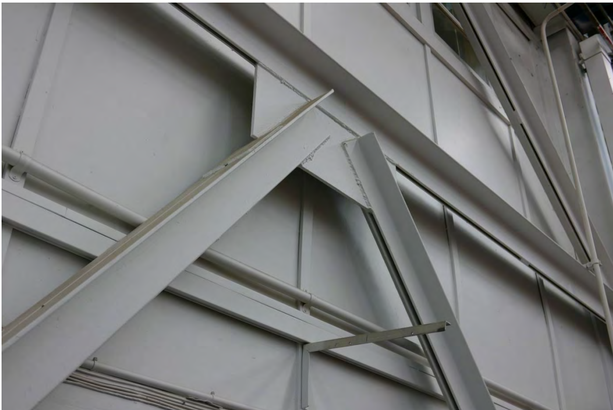
Plate 8 Structural welded RSJ triangulated detail Hangar 76 - image 795
