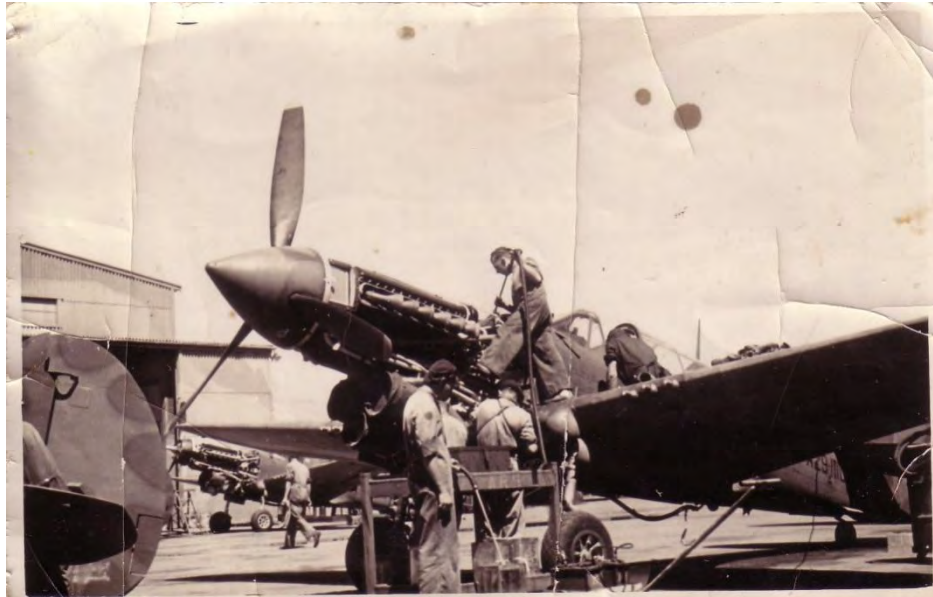
Plate 10 RAAF Base Amberley re-fuelling Kittyhawk with Bellman Hangar in background (Source J. Nelson)
