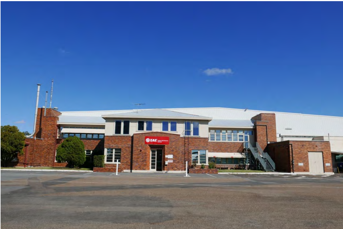
Plate 6 Hangar 76 square front elevation – image 705
