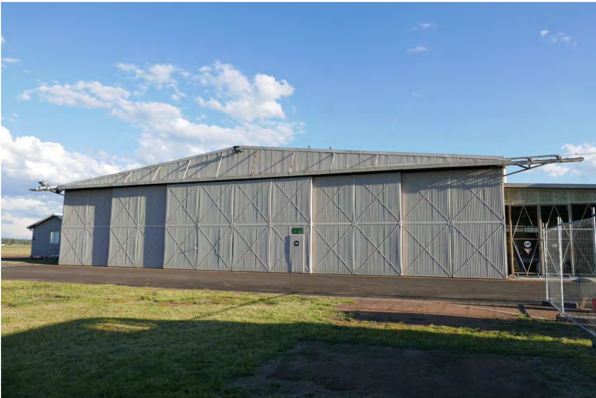
Plate 10 Hangar 258 north elevation – image 10306
