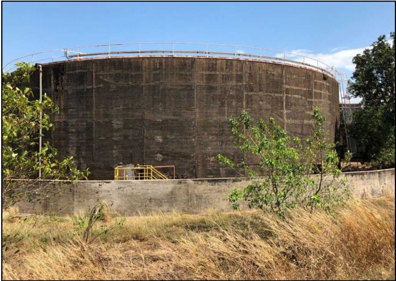
Image 3: One of the six above-ground storage tanks currently on the site
