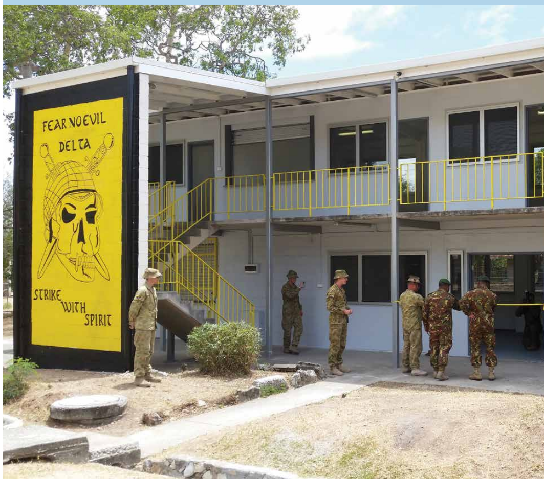
Defence Cooperation Team Leader, Lieutenant Colonel Shaun Fletcher, and Commanding Officer 1st Royal Pacific Islands Regiment, Lieutenant Colonel Napyo, opening the newly refurbished D Company headquarters building at Taurama Barracks, Port Moresby. The building was refurbished under Exercise Puk Puk.
