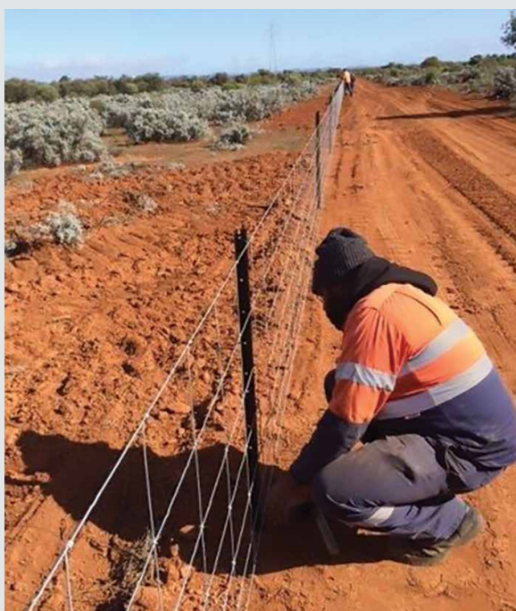
Walga Mining and Services employee installing perimeter fencing and security signage at the expanded Cultana Training Area.
