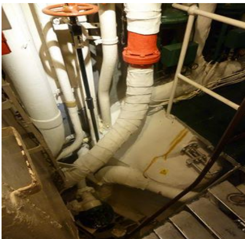
Asbestos lagging on board a vessel.
