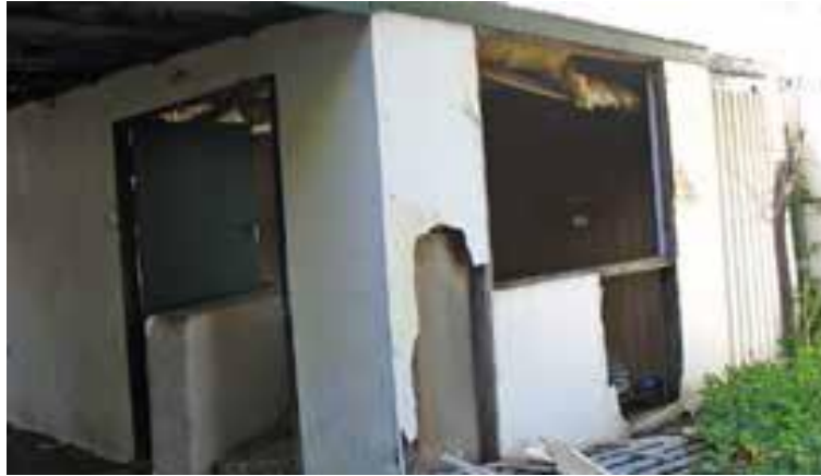
Broken asbestos cement sheets in old buildings.
