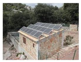
Figure 4 - Small Roof mounted Array
