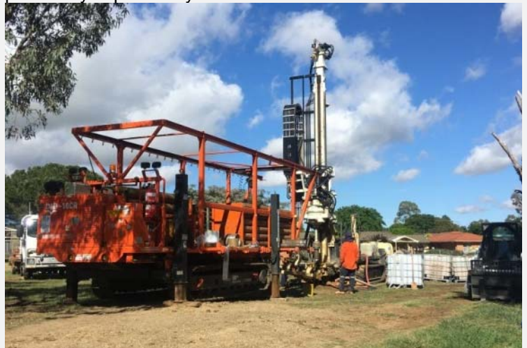
Drill rig used to install groundwater bores
