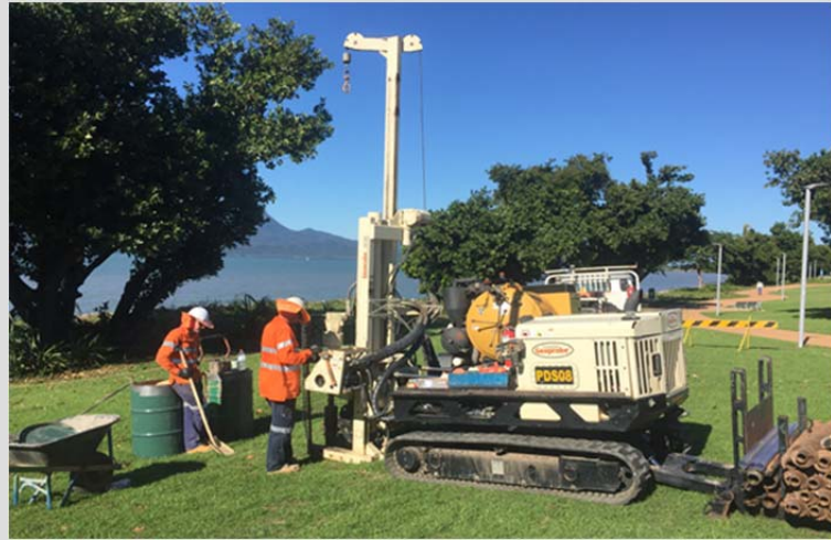
Small rig used to drill boreholes
