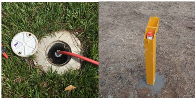
Ground-water monitoring wells, flush mount (left) and protruding (right)
