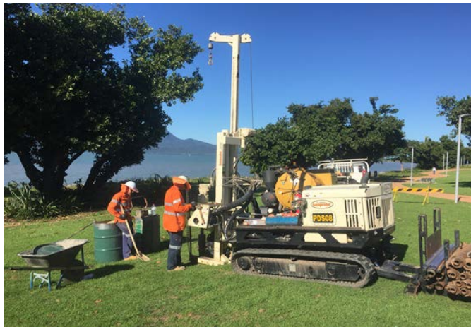
Small drill rig used to develop boreholes
