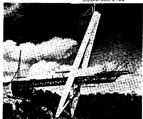
Above: Picture shows the key A-frame in position and at bottom how it supports the bridge's main span.
