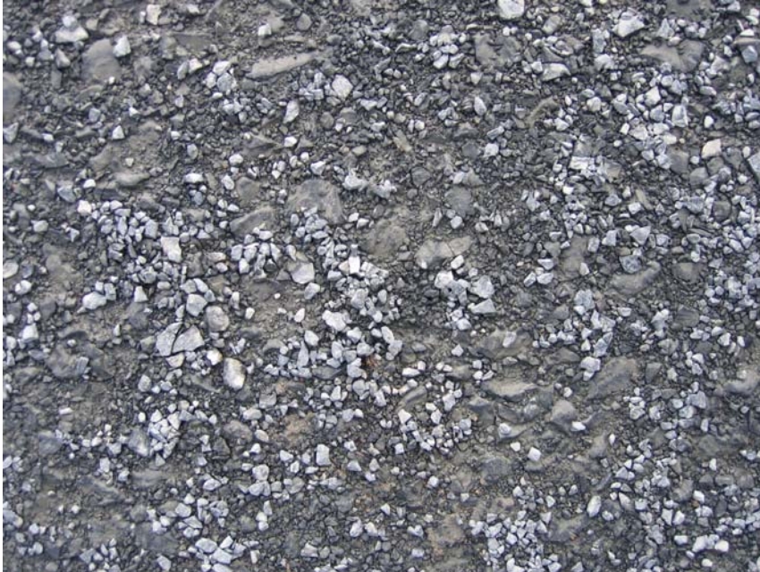
Photograph 7. Surface before rolling.
