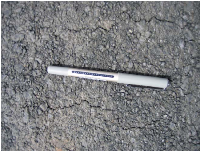
Photograph 8. Surface after rolling.
