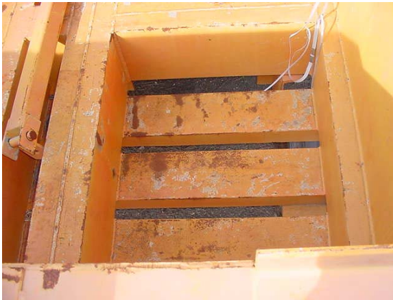
Front right ballast box
