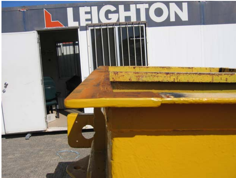
Photograph 9. Replaced steel plates.
