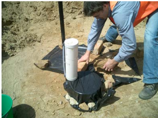
Plate1: Ring Infiltrometer testing on the surface of the Upper Shepparton clays.
