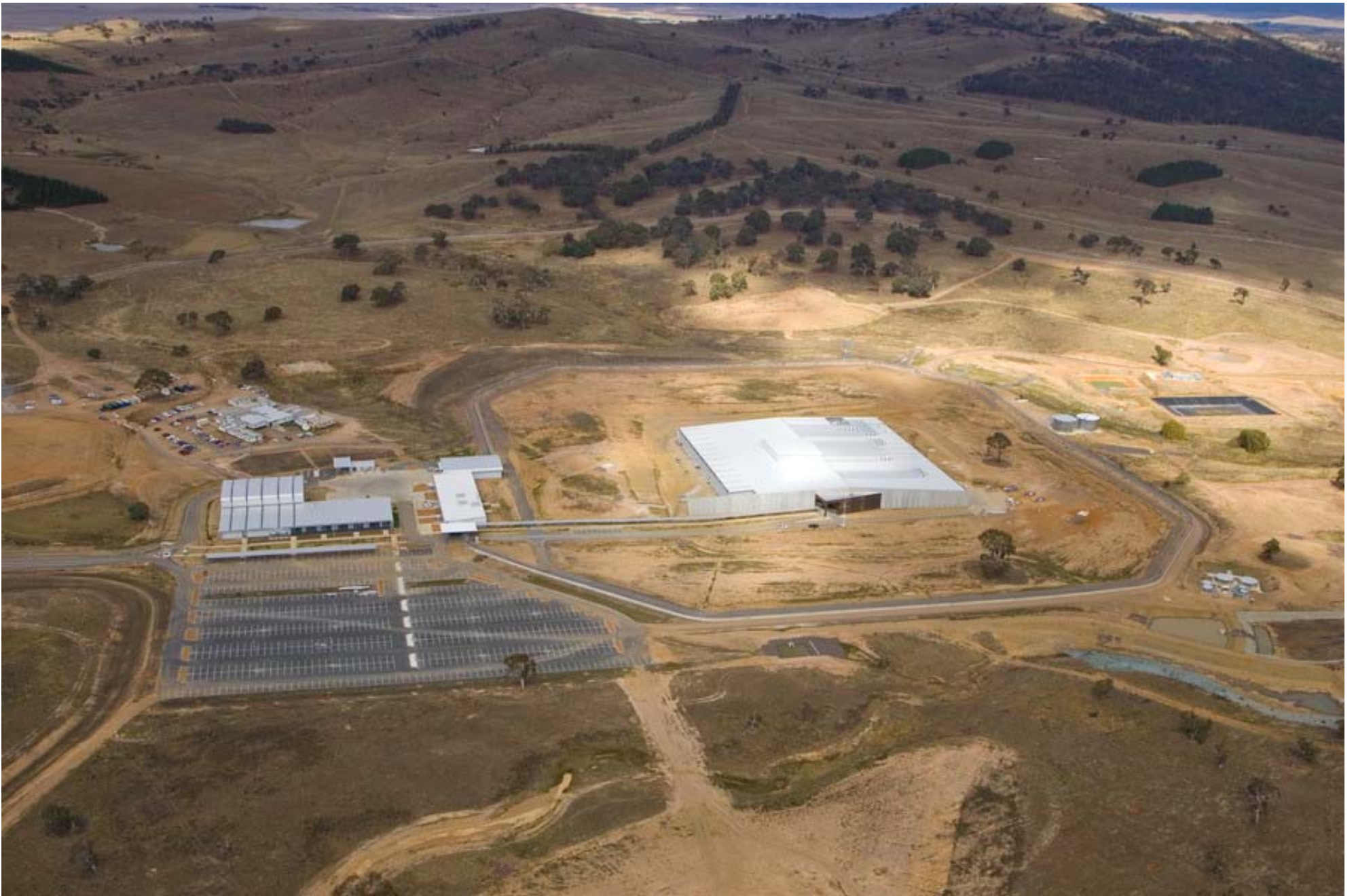
24 April 2008 – Headquarters (right) and support buildings
