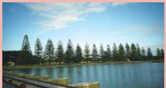
One of the Murray Barrages
