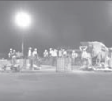
Night work to place concrete on runway at RAAF Amberley
