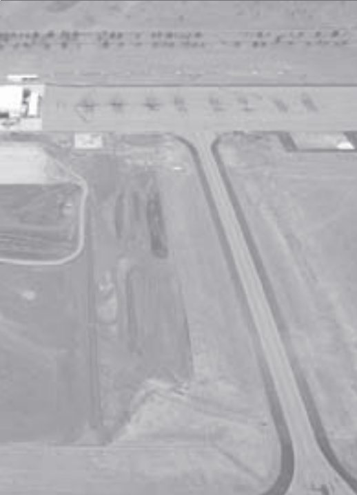
Air to ground photograph of RAAF Amberley base redevelopment
