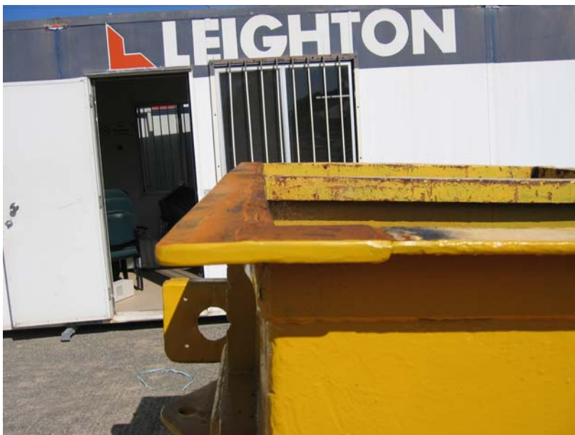
Photograph 9. Replaced steel plates.
