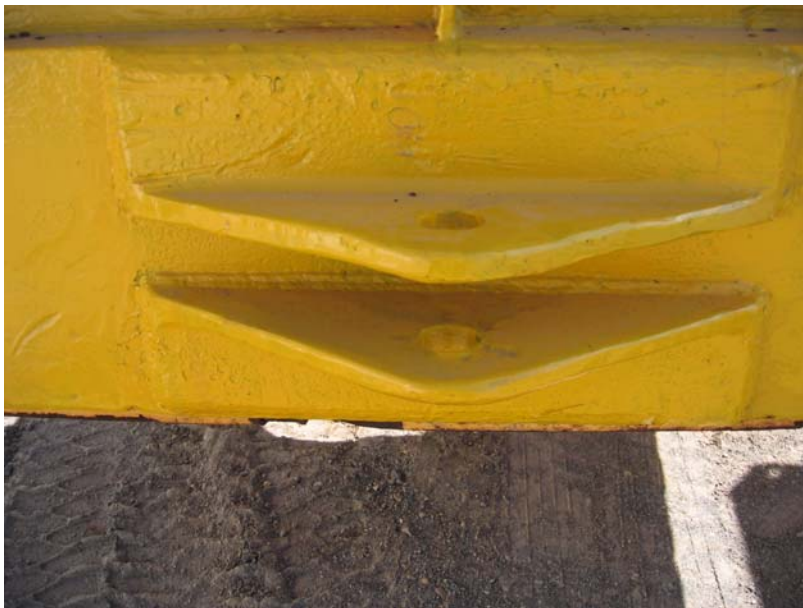
Photograph 7. New rear flanges.
